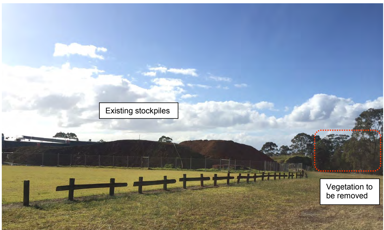
Photo 4: Existing site of the proposed activity
