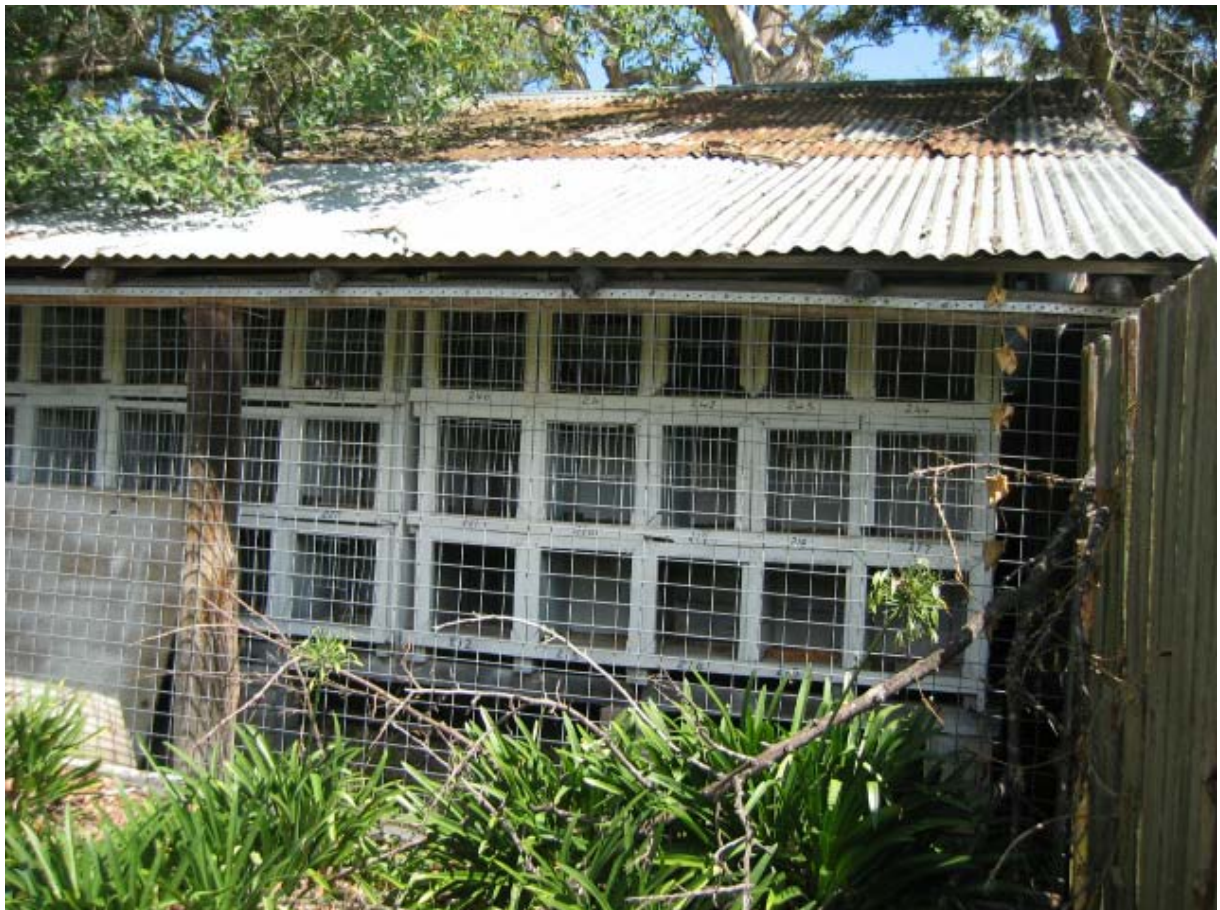
Figure No.B56: Poultry Pavilion, north elevation.
