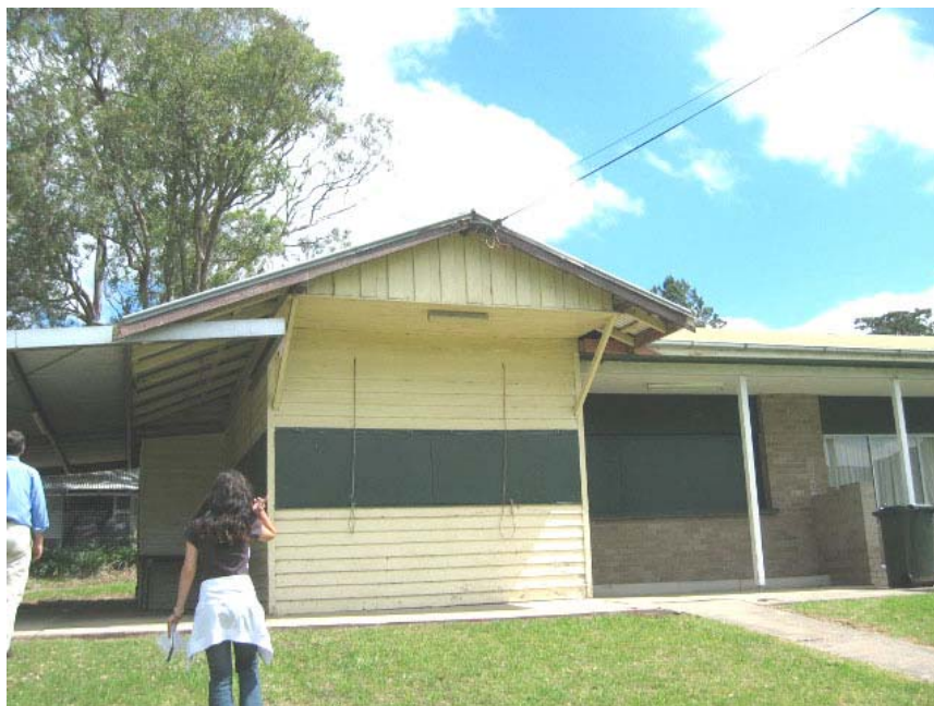
Figure No.50: Bar external.
