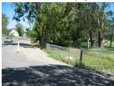
Figure No.31: East entrance and southern boundary fence.
