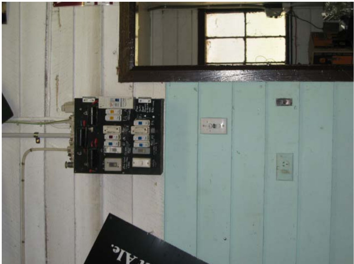
Figure No.B52: General view of bar interior. Figure No.B53: General view of bar interior.
