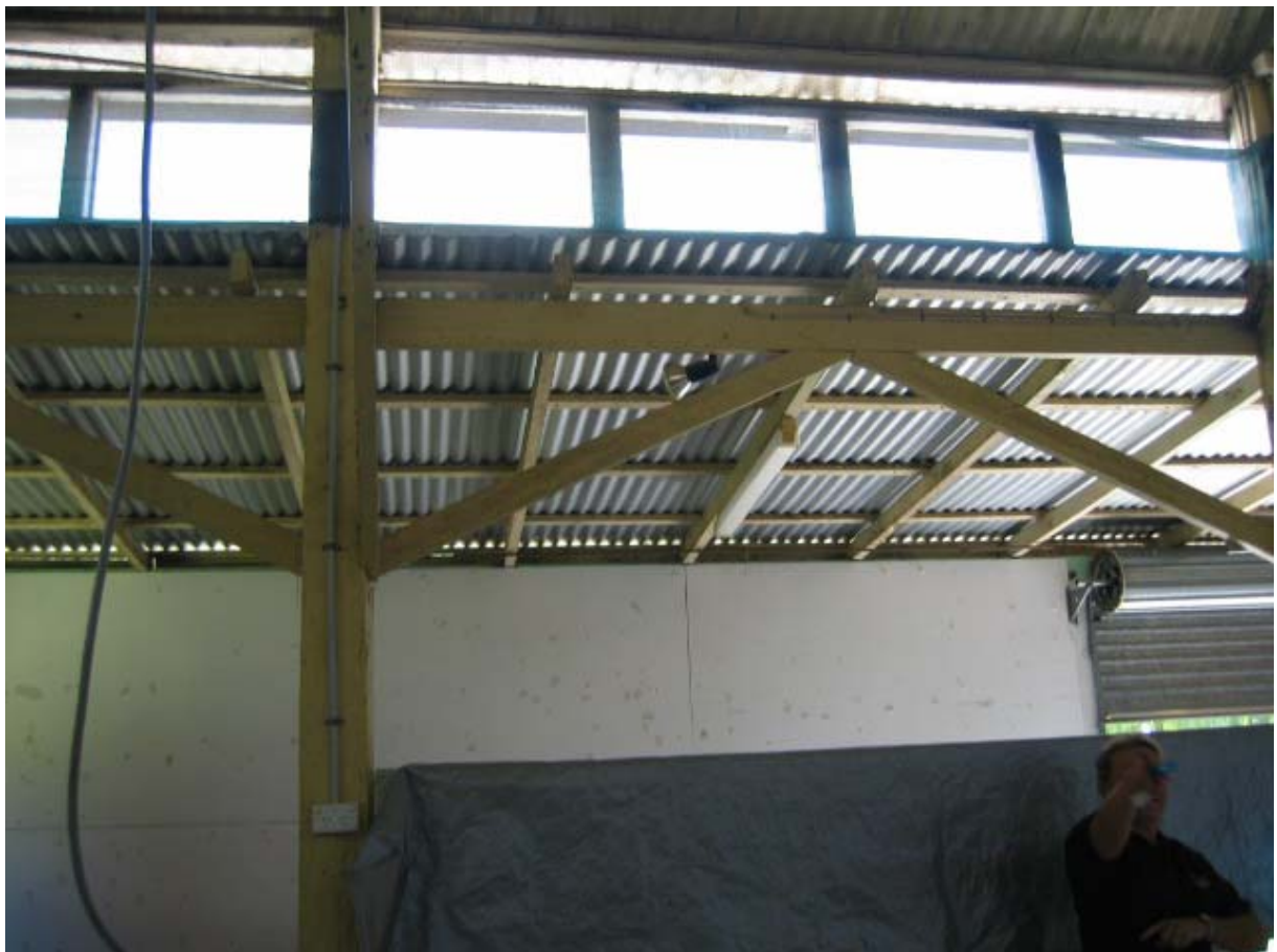
Figure No.B32: Agricultural Pavilion interior showing trusses and roof.
