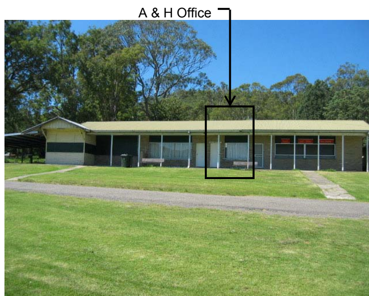
Figure No.45: Buildings from left to right: Covered area and bar, A & H Committee room, A & H Office and the kiosk.
