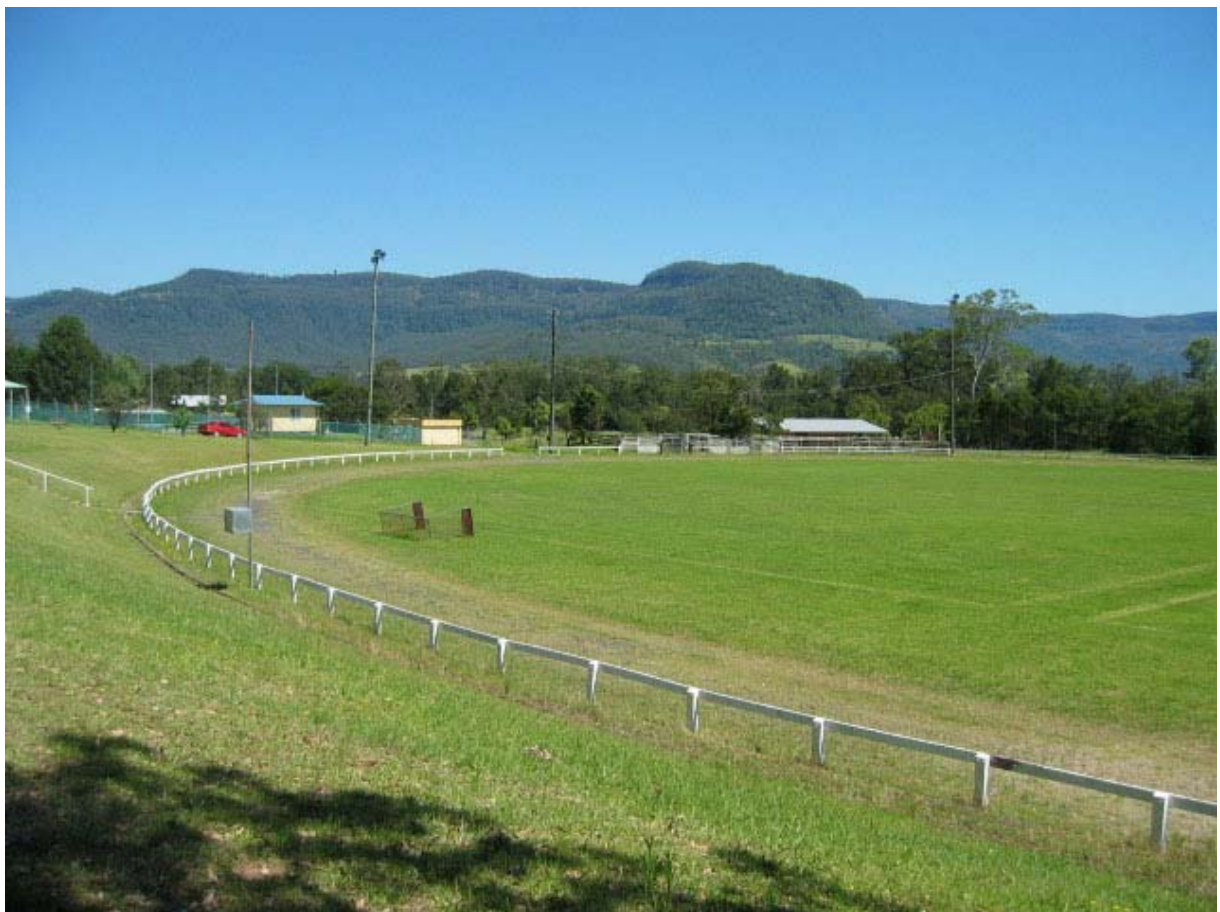
Figure No.B64: Showground ring and seating. Figure No.B65: Showground ring looking west.
