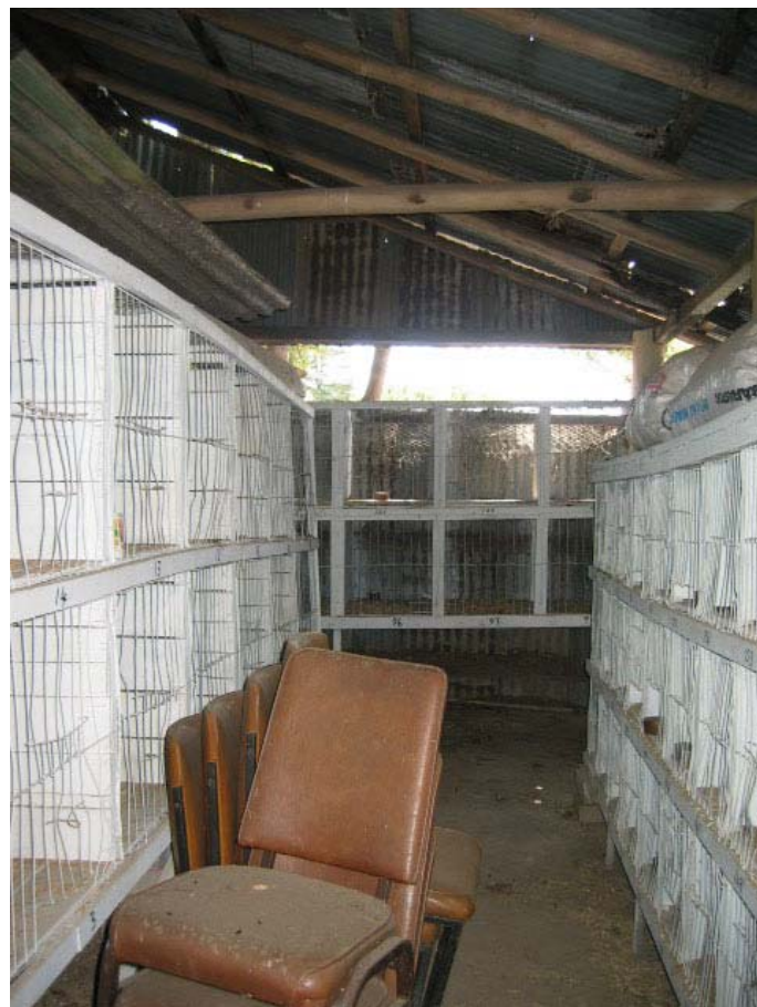
Figure No.B58: Poultry Pavilion, south elevation. Figure No.B59: Poultry Pavilion interior.
