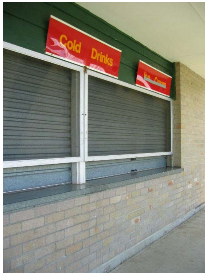
Figure No.B38: Recent buildings, including the bar, A & H rooms, the kiosk. Figure No.B39: Exterior of the kiosk.
