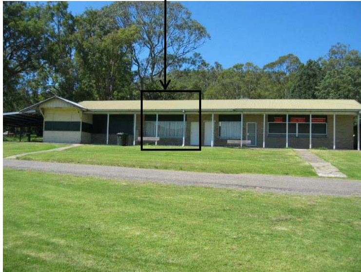
Figure No.48: Buildings from left to right: Covered area and bar, A & H Committee room, A & H Office and the kiosk.
