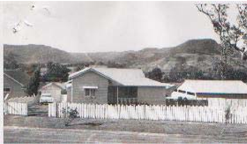
Figure No.7: Caretaker's Cottage, 1972.
