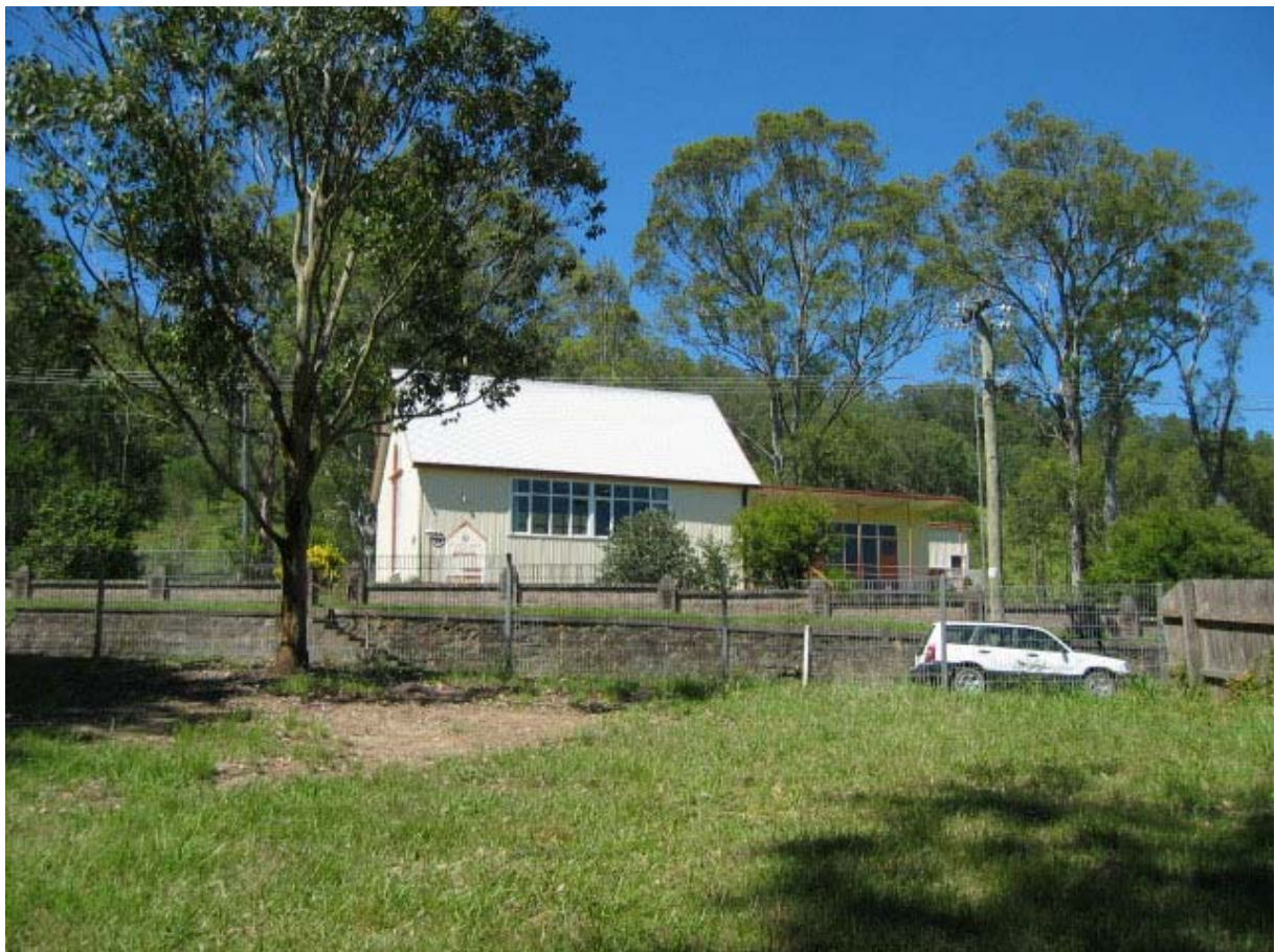
Figure No.B3: East elevation of the School of Arts building, as viewed from the carpark of Osborne Park.
