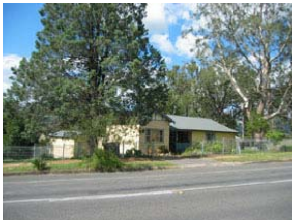
Figure No.53: Caretakers Cottage, front elevation.
