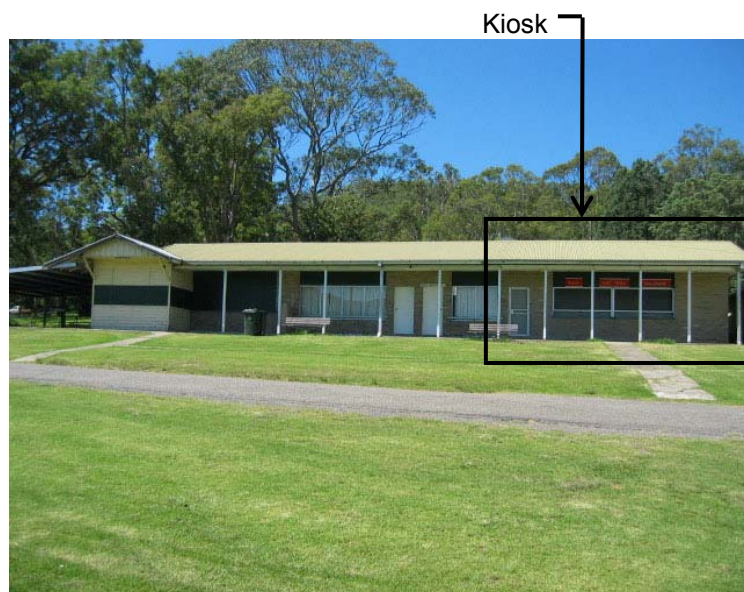
Figure No.41: Buildings from left to right: Covered area and bar, A & H Committee room, A & H Office and the kiosk.
