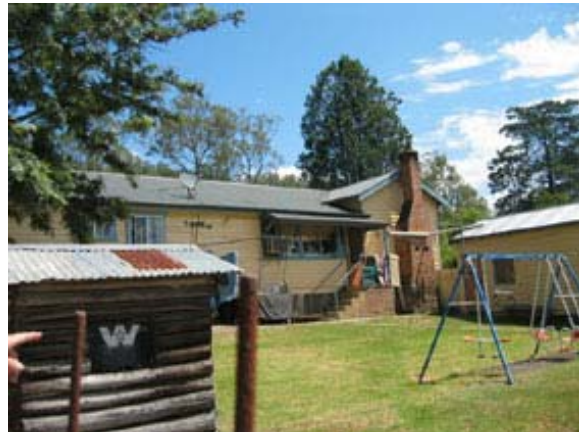
Figure No.54: Caretaker's Cottage, rear elevation.
