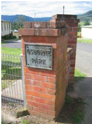
Figure No.62: Entrance piers.
