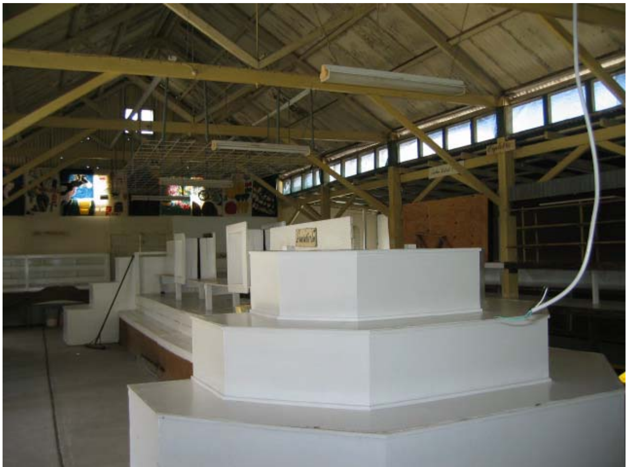
Figure No.B26: Sign above the no longer used northern entrance door to the Agricultural Pavilion.
