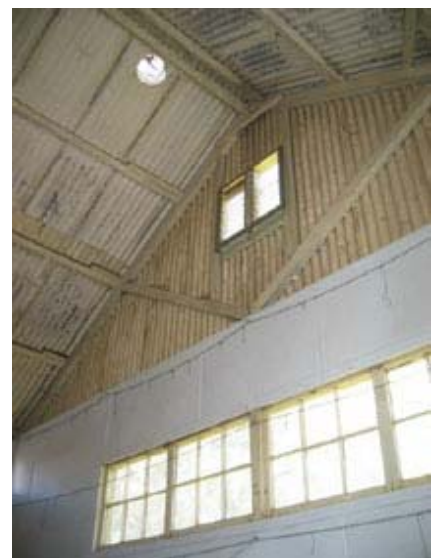
Figure No.22: Agricultural Pavilion interior.
