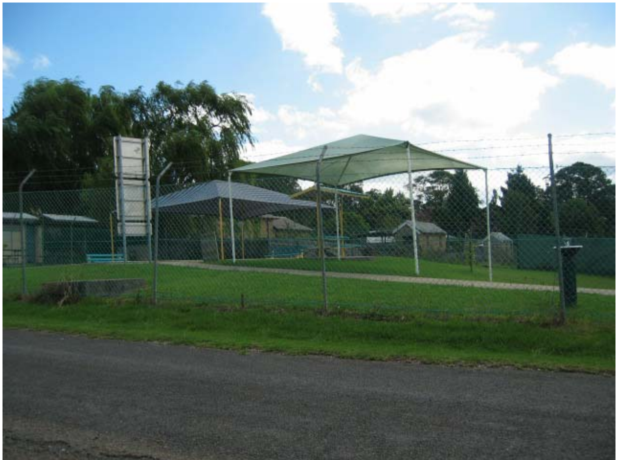
Figure No.B92: General view of the swimming pool area. Figure No.B93: Shade structures over the swimming pools.
