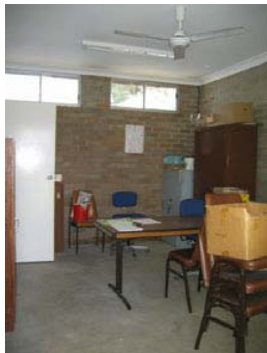
Figure No.47: Office interior looking north.
