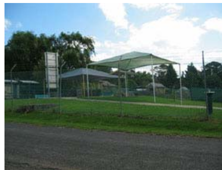
Figure No.58: Swimming pools and shade structures.
