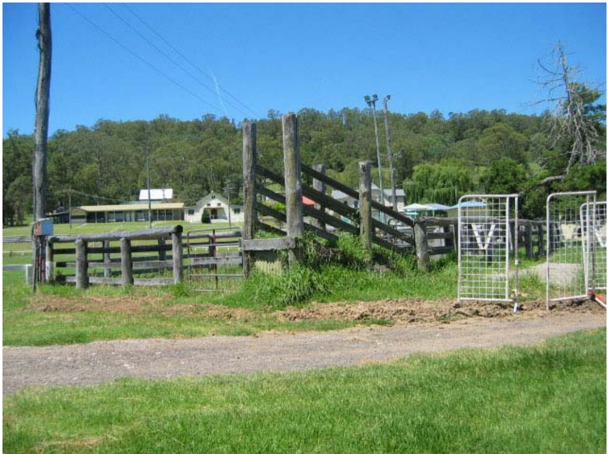
Figure No.B84: Horse stalls along the north elevation.
