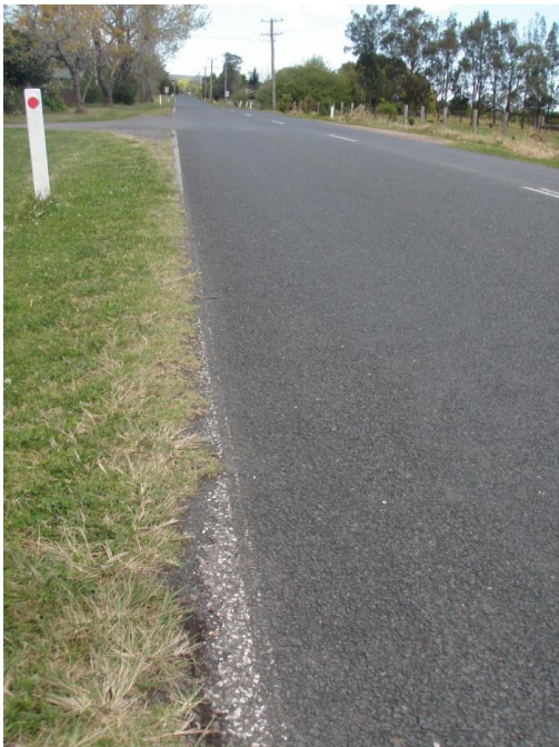
Photo 7: Example of the road shoulder on Terara Road disappearing weed invasion / Minimal road shoulder on the Princes Highway
