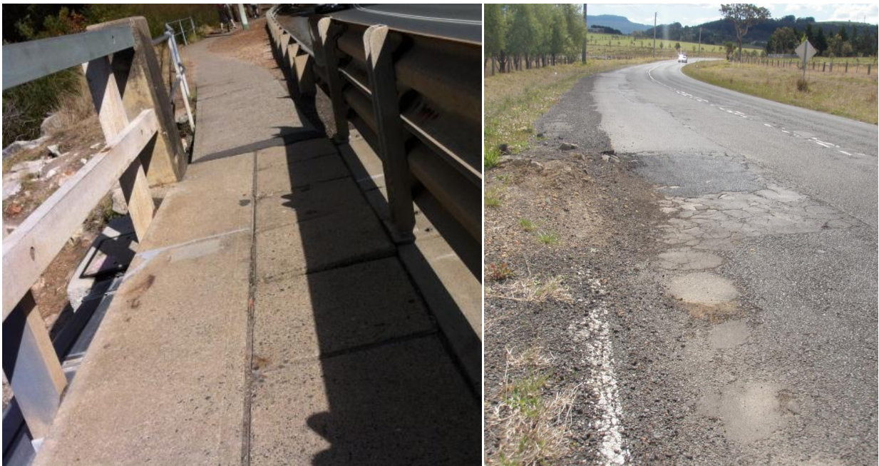
Photo 6: Example of squeeze point at Moona Moona Creek Bridge and a failing road shoulder on Coolangatta Road
