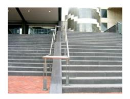
Handrails should not encroach the minimum width of pathways, ramps, step ramps and stairways.
