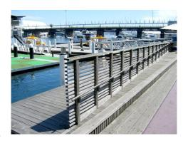
Continuous handrails should be provided on both sides of all ramps or stairs.
