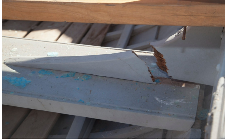
Broken timber in the boat
