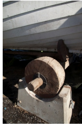
Note shape & good condition of timber wheels and concrete stays.
