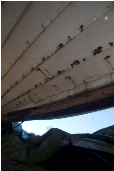
Note the paint cracking
