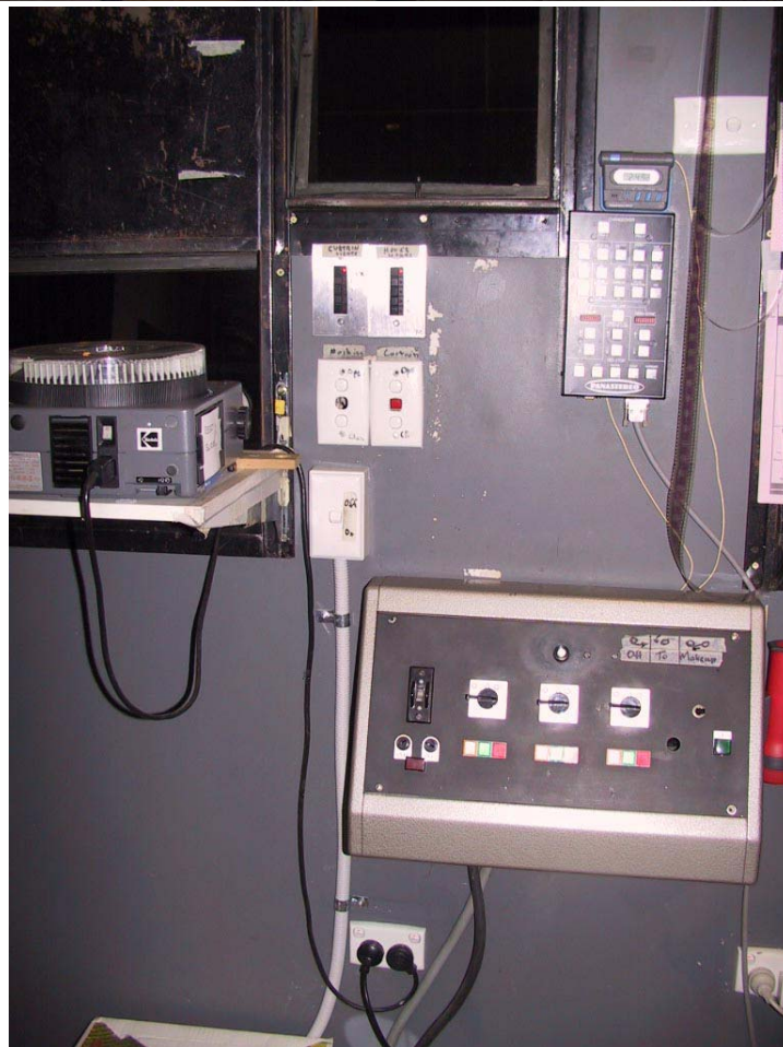
Figure No.41: Projection room (south wall).
