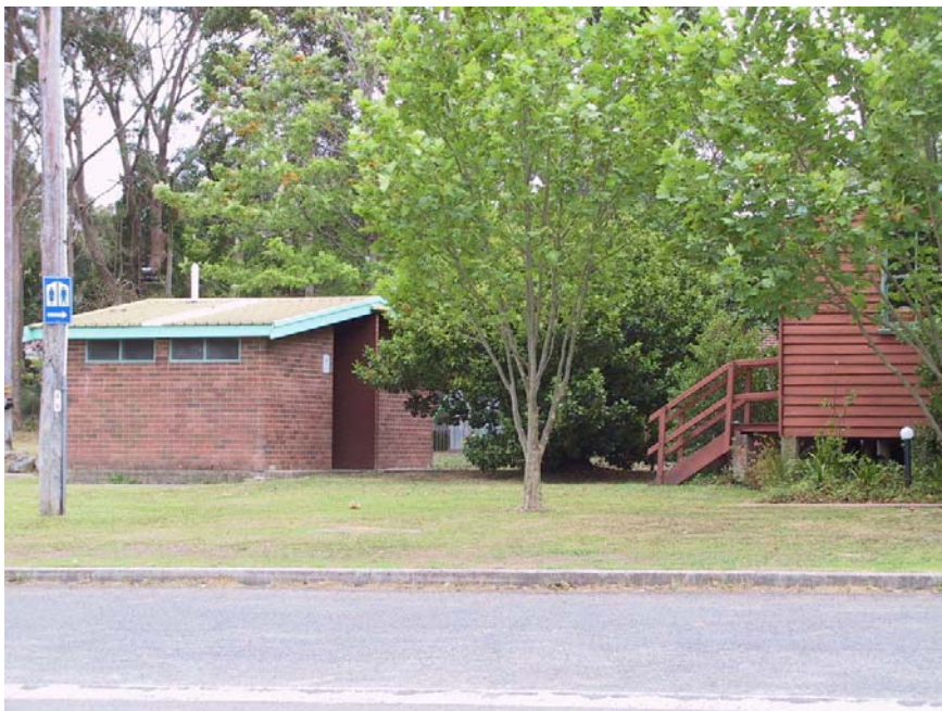
Figure No.11: Toilet block to rear of subject building.
