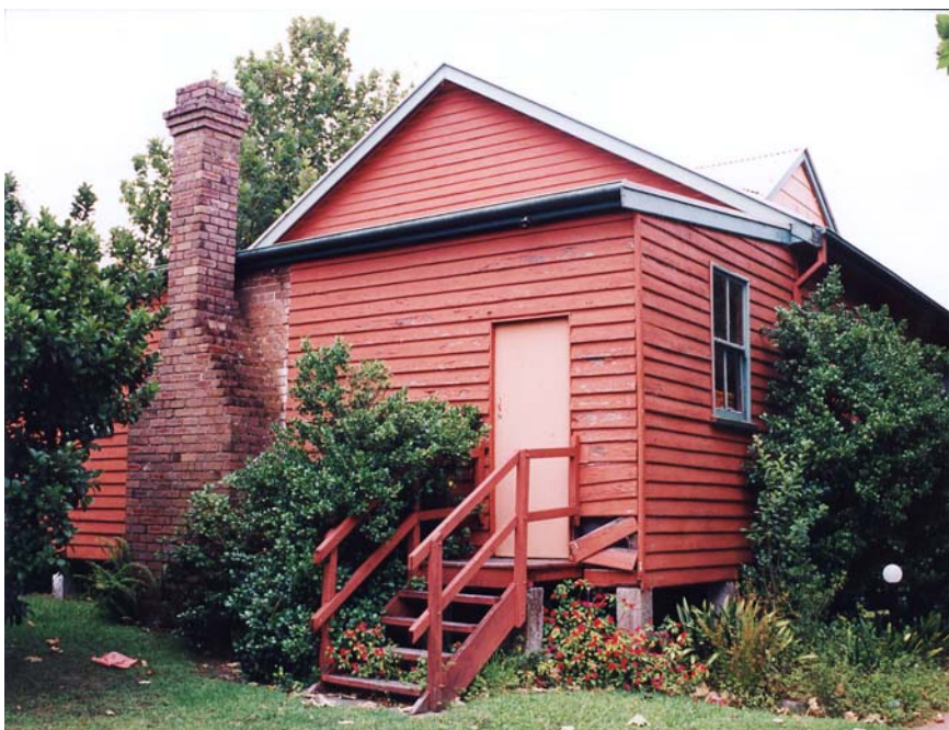
Figure No.13: Rear elevation of subject building.
