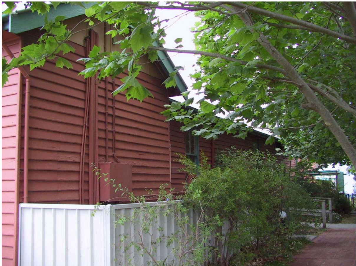
Figure No.13: View down north side of subject building.
