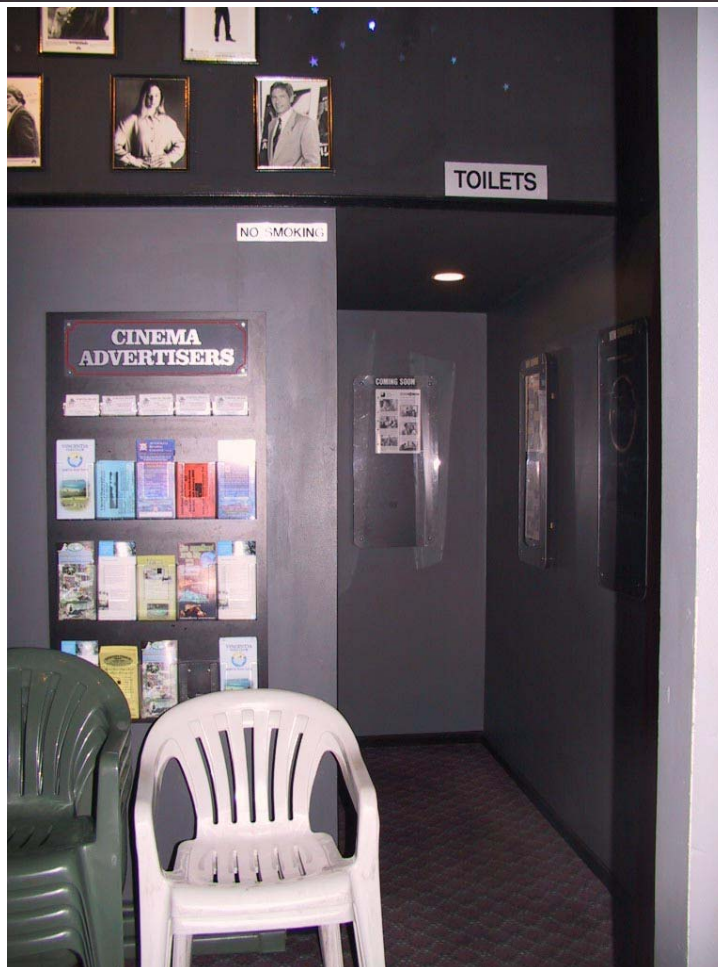
Figure No.25: Original timber panel ceiling and vent in foyer.
