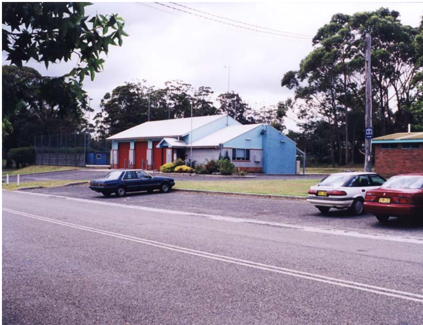
Figure No.10: Huskisson Fire Station.
