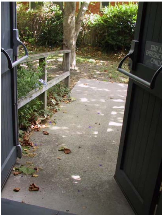
Figure No.26: Disabled Access/exit along northern elevation.
