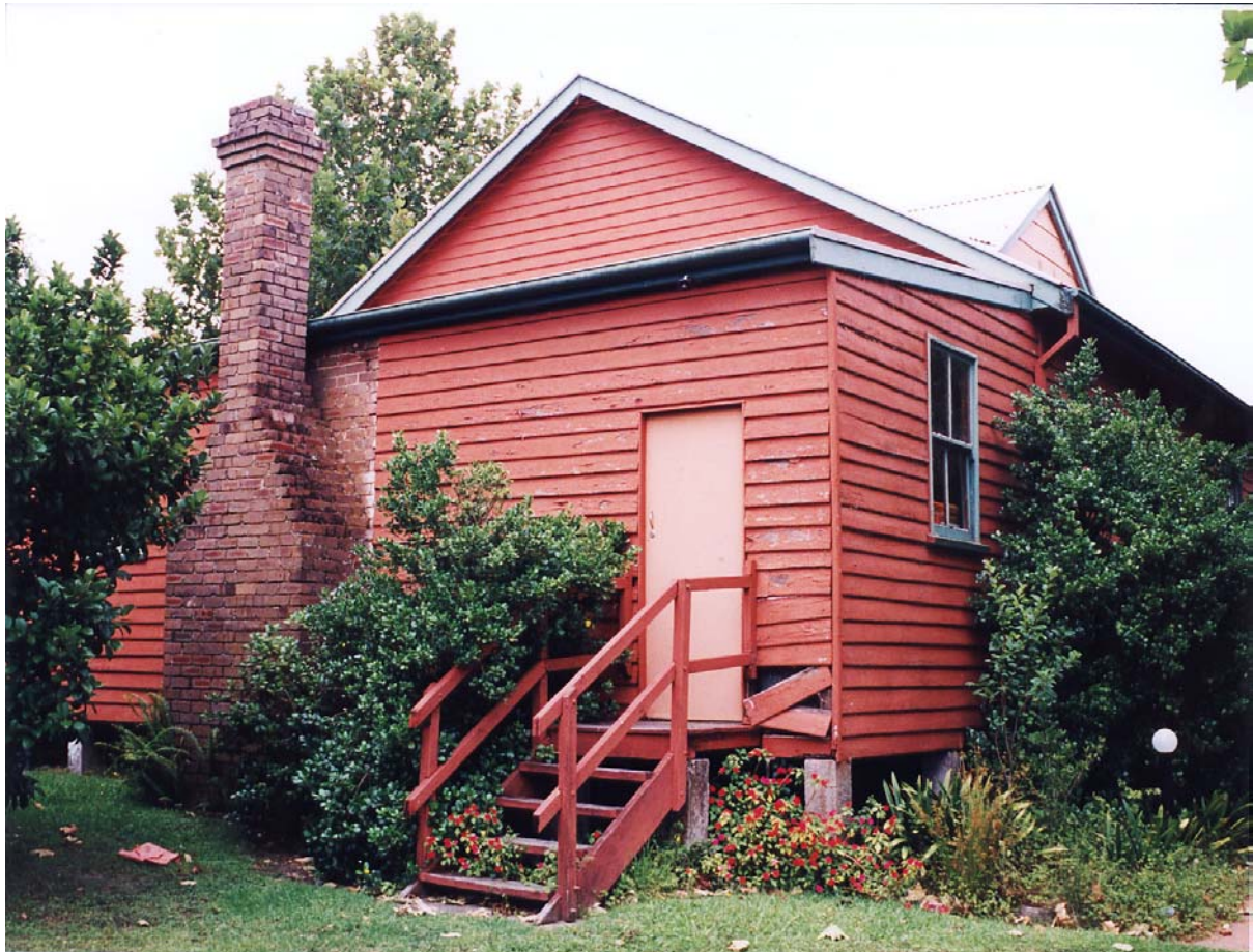
Figure No.9: Front and part side elevation of subject building.
