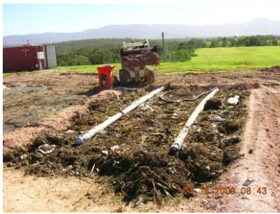
1 st Step 2x HDPE air pipes
