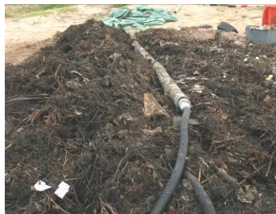
2 nd Step HDPE pipes in core
