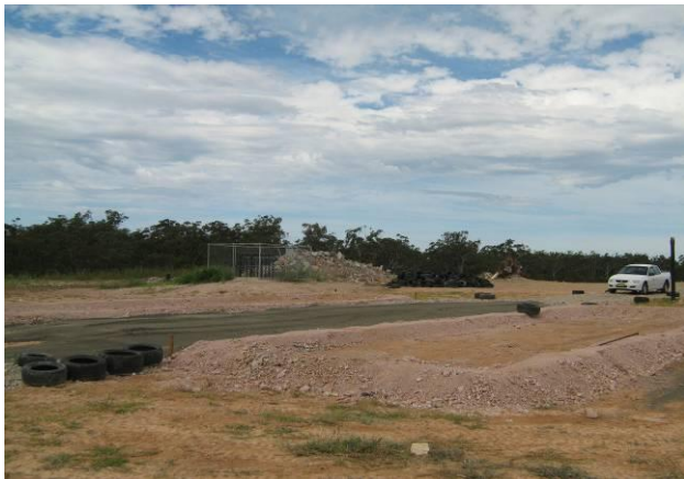
Composting bay with all weather service roads
