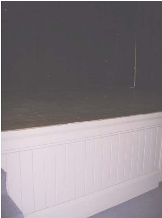
Figure No.21: Timber board detailing on base of stage.
