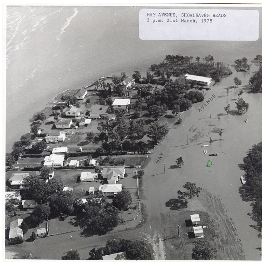
Photograph 2: Hay Avenue, Shoalhaven Heads - March 1978 Flood
