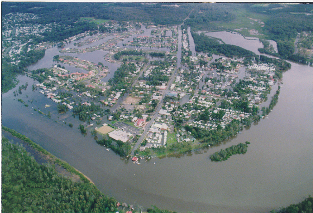
SUSSEX INLET - JUNE 1991 FLOOD
