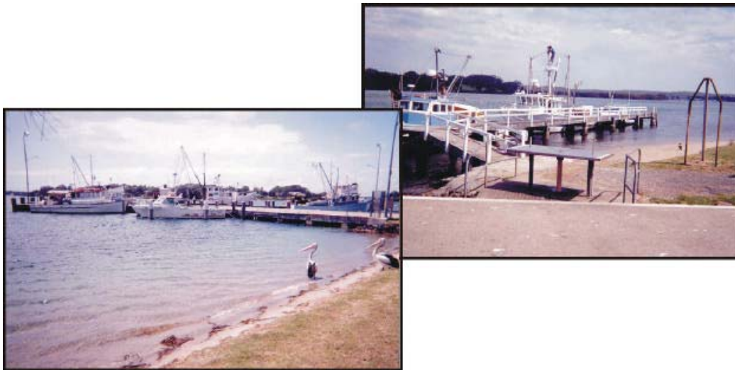
Figure 13. Greenwell Point Fishermen's Wharf – on the left is the main wharf and on the right the old wharf (from Greenwell Point Waterway Facilities Needs Assessment. Webb, McKeown & Associates Pty Ltd, 2003).
