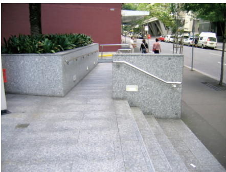
Building access ramp with adjacent stairs
