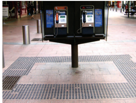
TGSI to alert people who are blind or vision impaired to pending obstacles.
