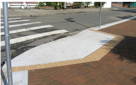
Kerb Ramp for pedestrian crossing
