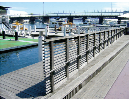
Access Ramp to wharf
