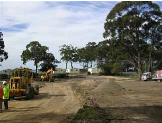
Huskisson Beach Tourist Resort Commencement of Earthworks
