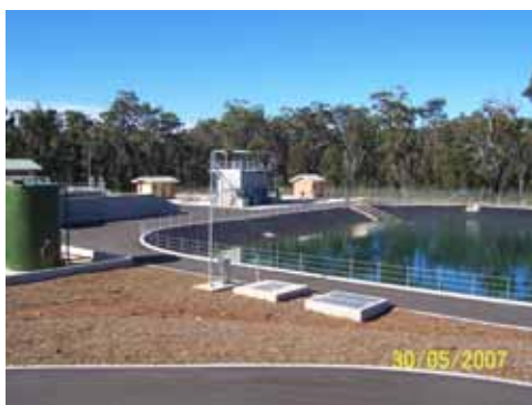
Conjola Treatment Plant
