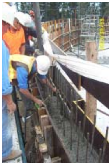
Bewong Reservoir – Pouring Wall concrete
