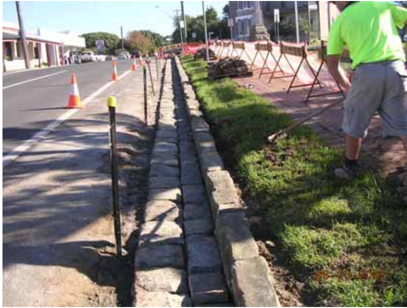
Princes Highway, Milton. Reconstruction of sandstone kerbing.
