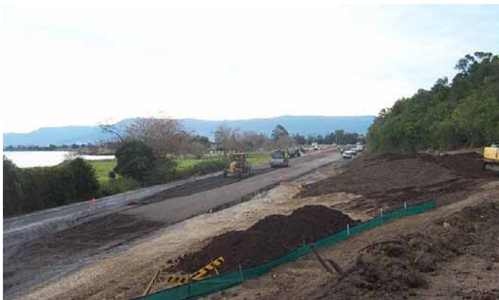
Bolong Road alignment and curve rectification
