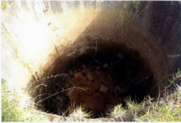
Figure 15 – old dome well with roof removed
