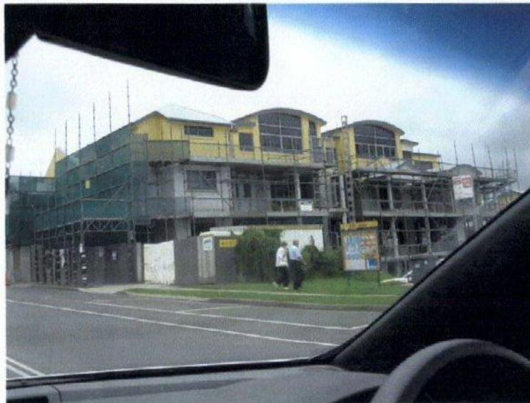
Figure. 13 - New 4 storey development under construction in Huskisson
