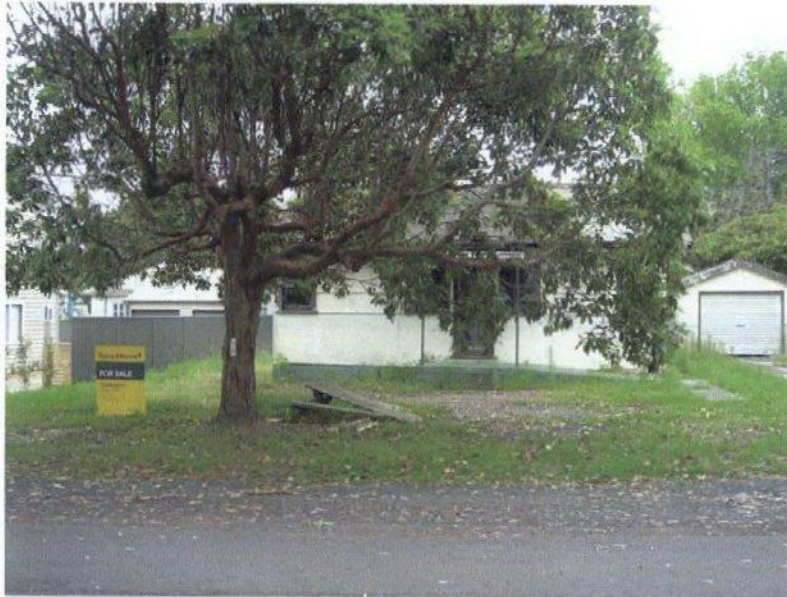
Figure. 15 - Street Elevation of existing dwelling at no. 19 Fegen Street, Huskisson (Fibro House, garage and all out-buildings to be demolished; tree to remain)
