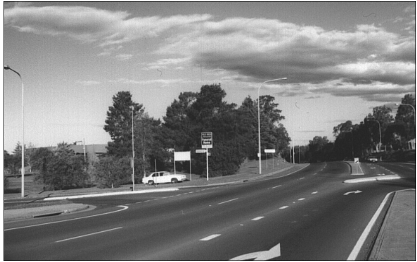
The Nowra bypass, 1998. The right turn gives access to Bridge Road. Graham Lodge is behind the pines in centre mid-ground.
