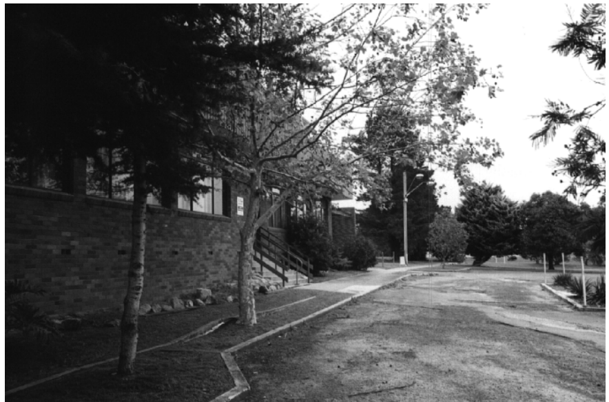
The eastern elevation with the former NBLC building in foreground. PF photograph 1998
