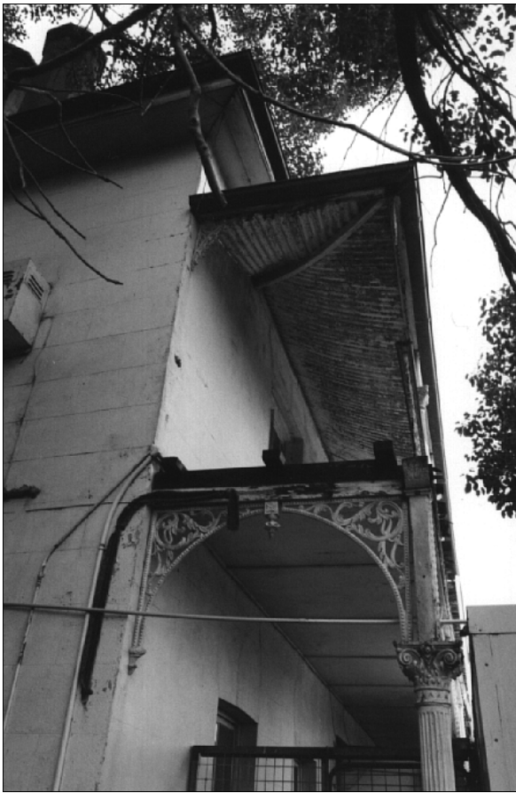
Top: Detailed photographs of the front verandah. Note the poor condition of the structure, and the adjacent [eastern] NBLC structure. Below: The eastern elevation. PF photographs 1998
