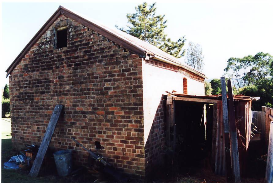
Figure 53 South elevation of cart shed and stables. Figure 54 South/ East corner of cart shed and stables. Note brickwork has shifted.
