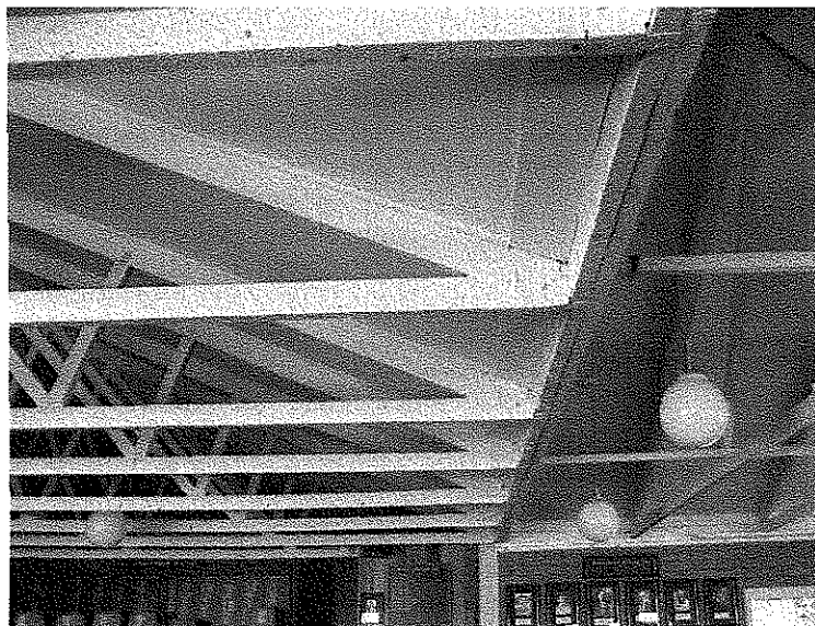
The existing function room structure.
