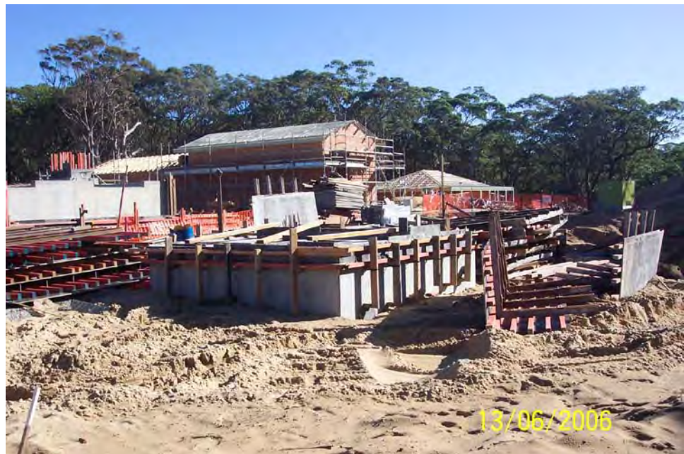
Conjola WWTP under Construction
