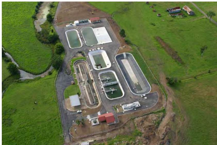
Aerial View of Berry Treatment Plant
