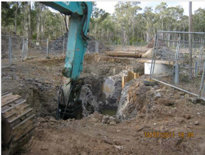
Nowra Park – laying 375mm DICL – Cancer Centre Main Diversion
