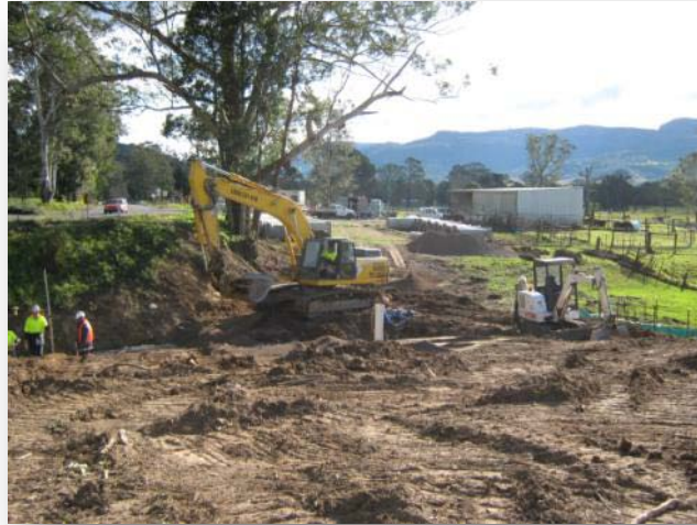
Access Road – Kangaroo Valley Preparation for Twin Cell Culvert Installation
