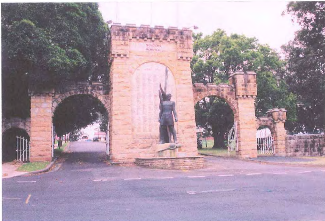
Fig. 5.24 - Inter-War Castellated Gateway viewed from West Street. Note staining to stonework at upper level and flanking fence.
