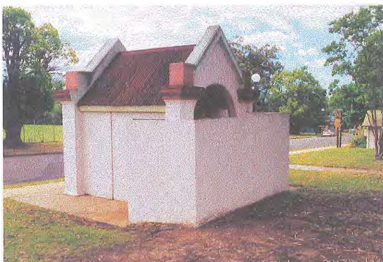
Fig. 5.19 - Victorian Masonry Gate and Toilet viewed from south western side showing added screen wall as part of the toilet conversion.
