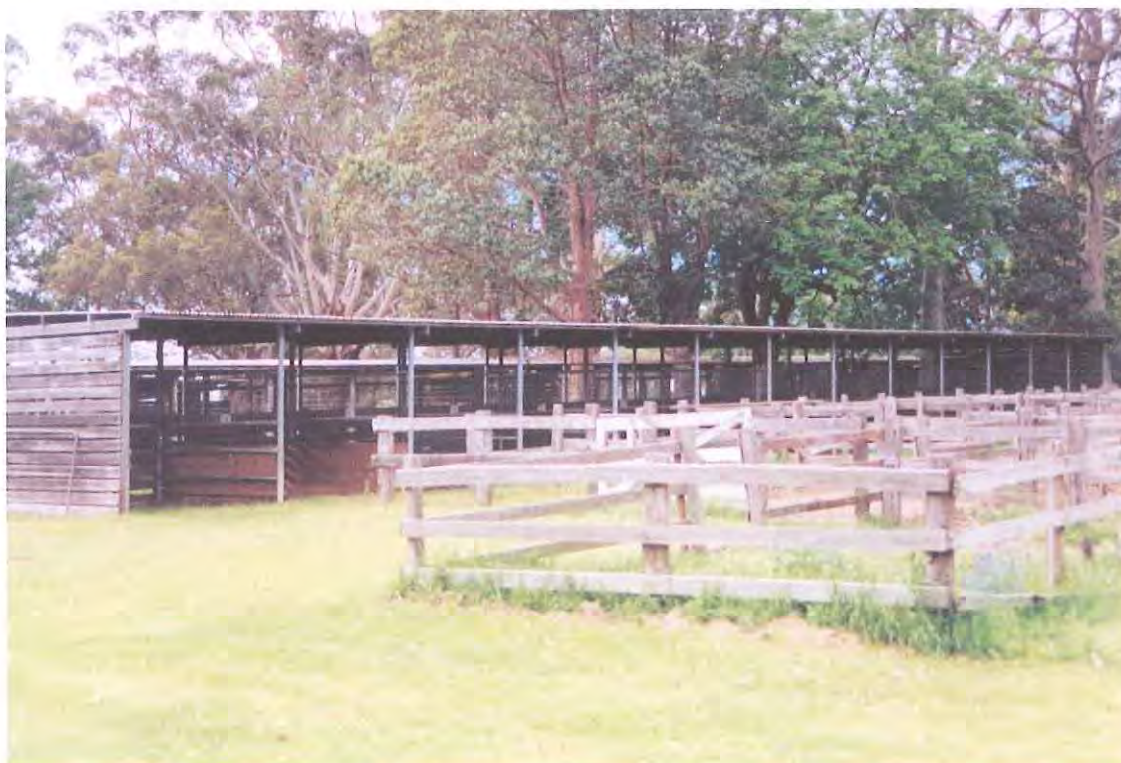
Fig. 5.34 Precinct 3 - showing typical timber and steel pipe framed stalls and timber post and rail fencing in foreground.
