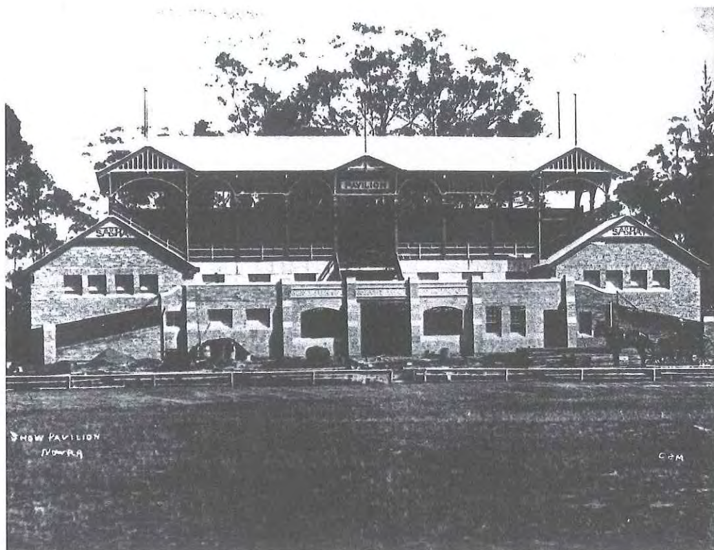
Fig. 5.10 - Federation Pavilion in original configuration. Note changes to gables of halls at either end and to side access stairways and podium.
