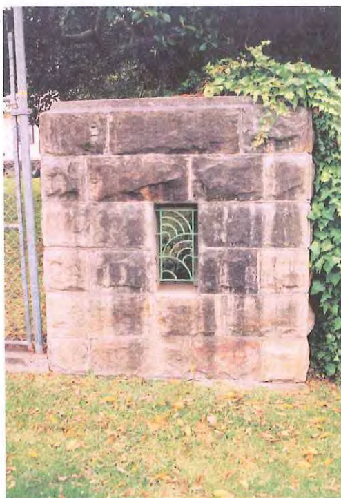
Fig. 5.25 - Detail of gateway showing decorative window in flanking fence. Note staining to ashlar stonework.
