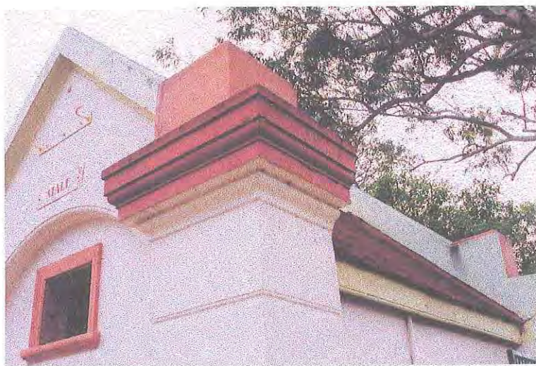
Fig. 5.20 - Detail of toilet showing cornice moulding and quoins formed in render at corners.
