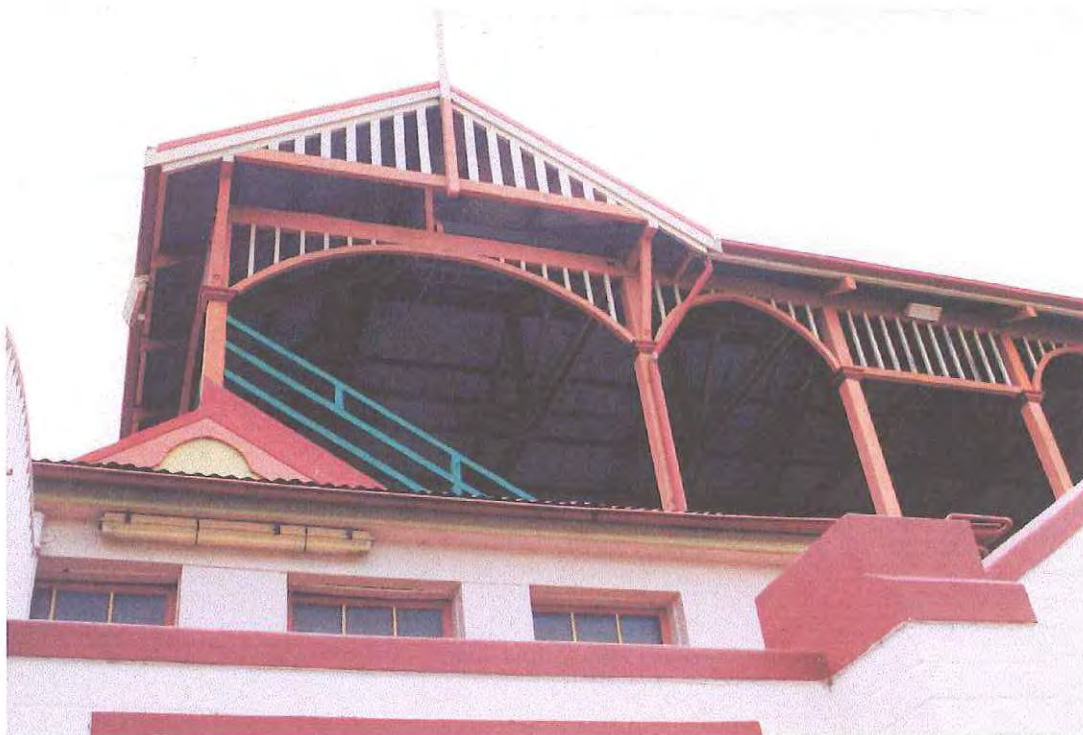
Fig. 5.13 - Detail of Federation Pavilion showing decorative timber work to gables.
