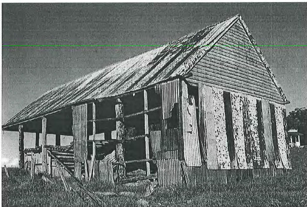
Above: Chaff cutting shed and fodder store on raised timber floor. Natural round timber post have been scorched in fire, sapling beams. Weather board gable, replacement sheet iron all cladding. Looking south MH 1997 photograph 2.21
