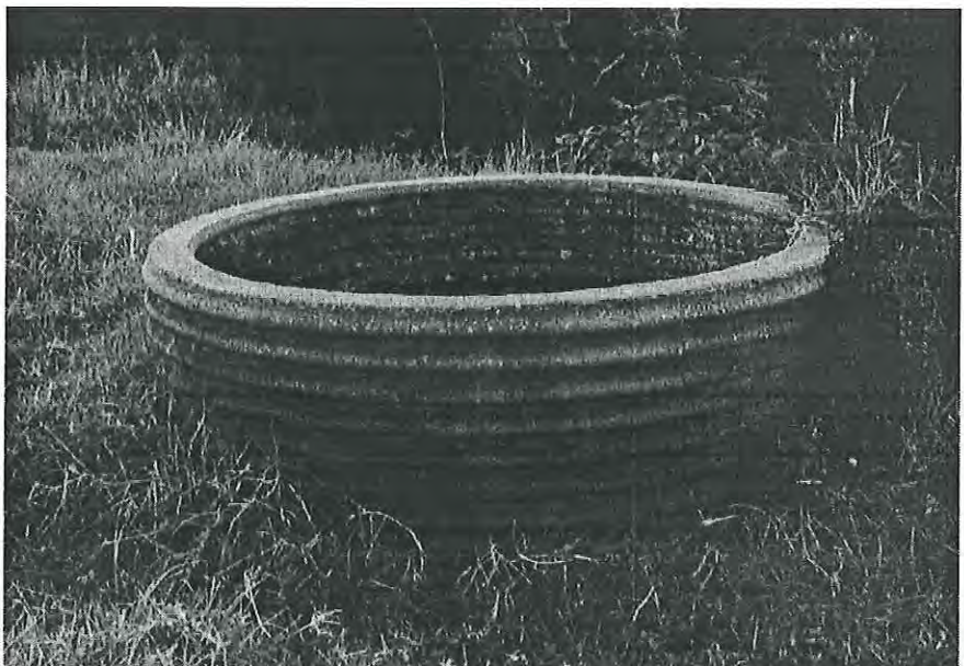
Water trough formed from concrete using corrugated iron formwork. MH 1997 photograph 14.9
