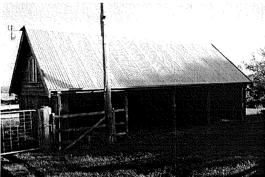
Walk through dairy, renovated. Southern rear wall filled in with recycled timber slabs. The pulley is still present for loft. Looking south MH 1997 photograph 1.5
