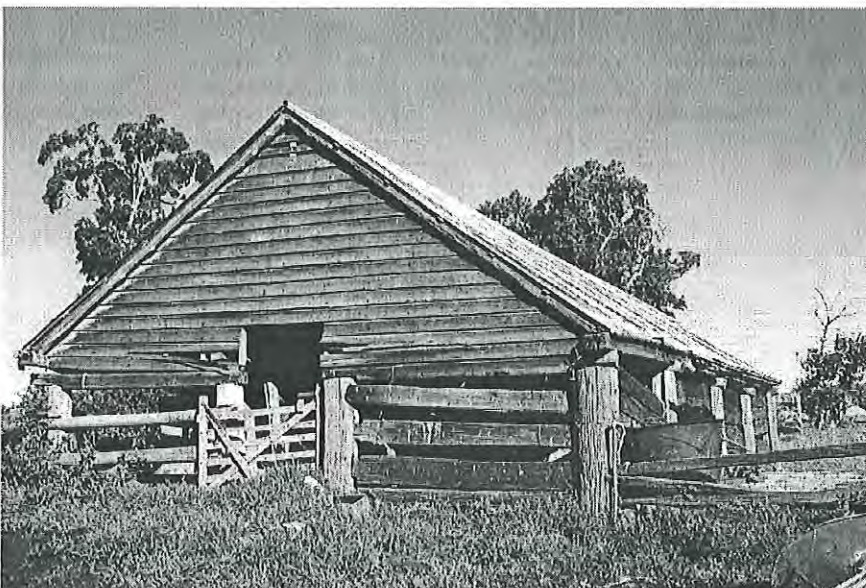
Pig sty northern weatherboard gable end, natural round posts, squared top plates, split timber horizontal slabs; western wall held in vertical grooves down length of posts (drop log construction). Tallow pot used as water trough. Looking south MH 1997 photograph 12.11
