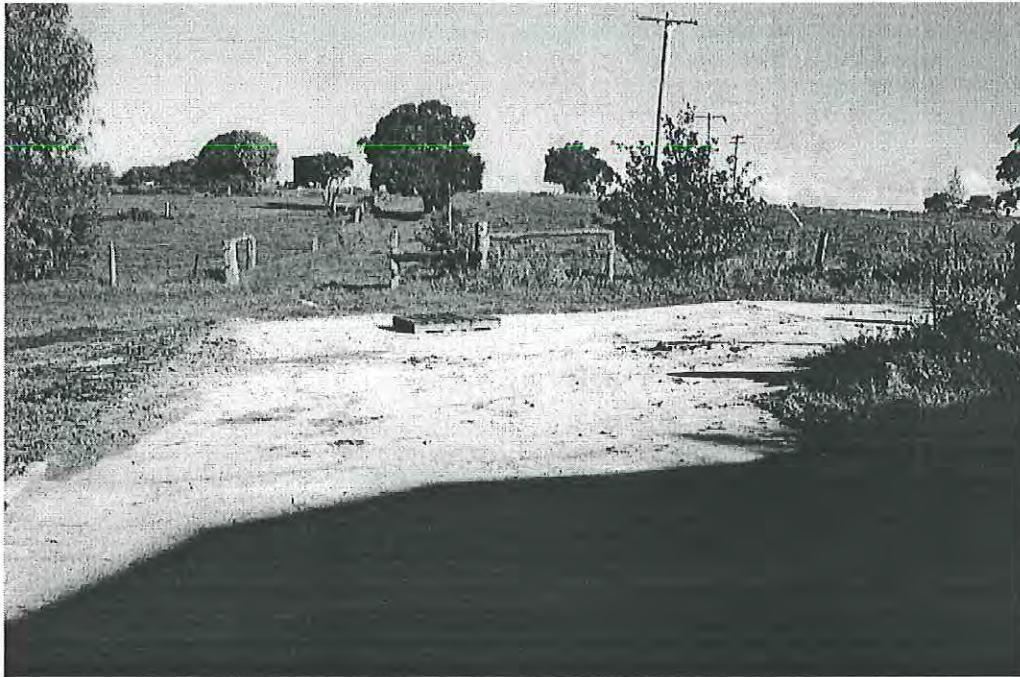
Above: Whoppindally, concrete base of earlier milking bails, 4 bails, dish drain along eastern edge, (LHS) cows entered from east. Former natural round timber post construction, post holes filled in. Distance shows lane way from paddock to this set of bails. Looking south. MH 1997 photograph 2.16
