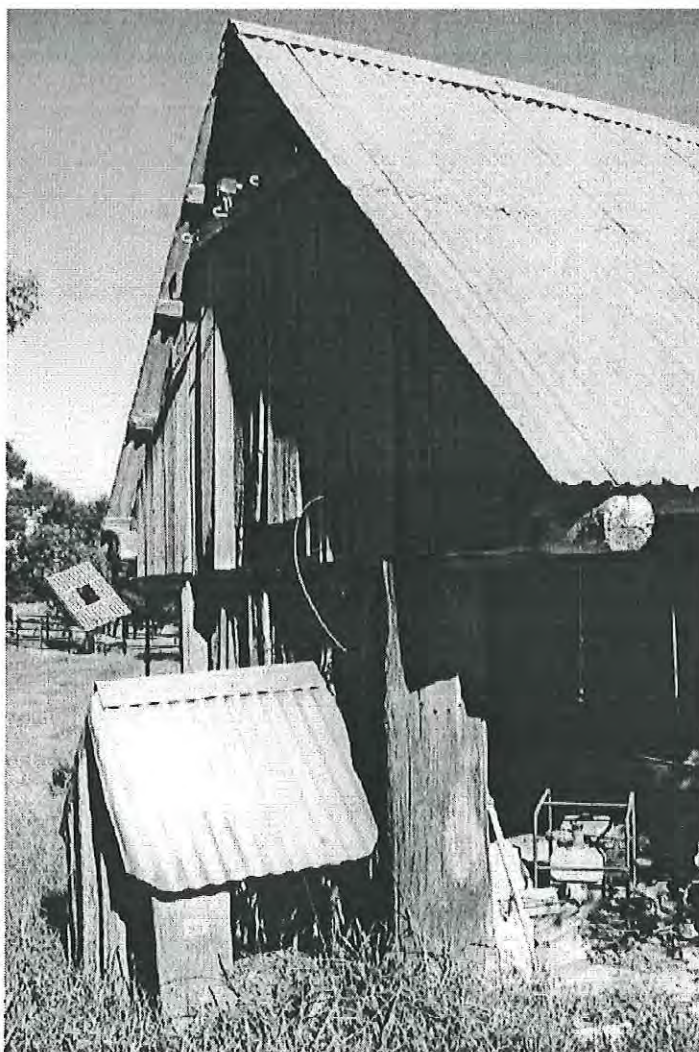
Right: Milking bails, detail natural round timber posts, split timber slab lower level, sawn timber boards, gable, corrugated iron roof. Looking south-west MH 1997 photograph 8.5
