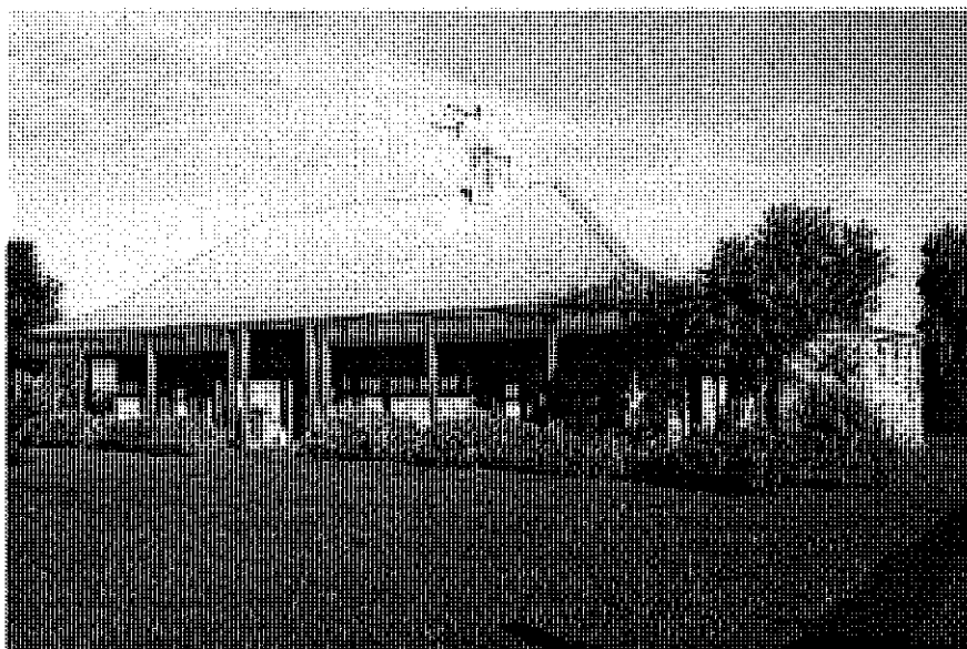
'Claydon Park' original stone section of house with stone rear extension, new timber verandah and new corrugated iron sheeting roof. Original roof was shingled. Metal tiles (Moorewood and Rogers, patented 1856) were on eastern hip of roof. Looking south-east. MH 1997 photograph 1.3
