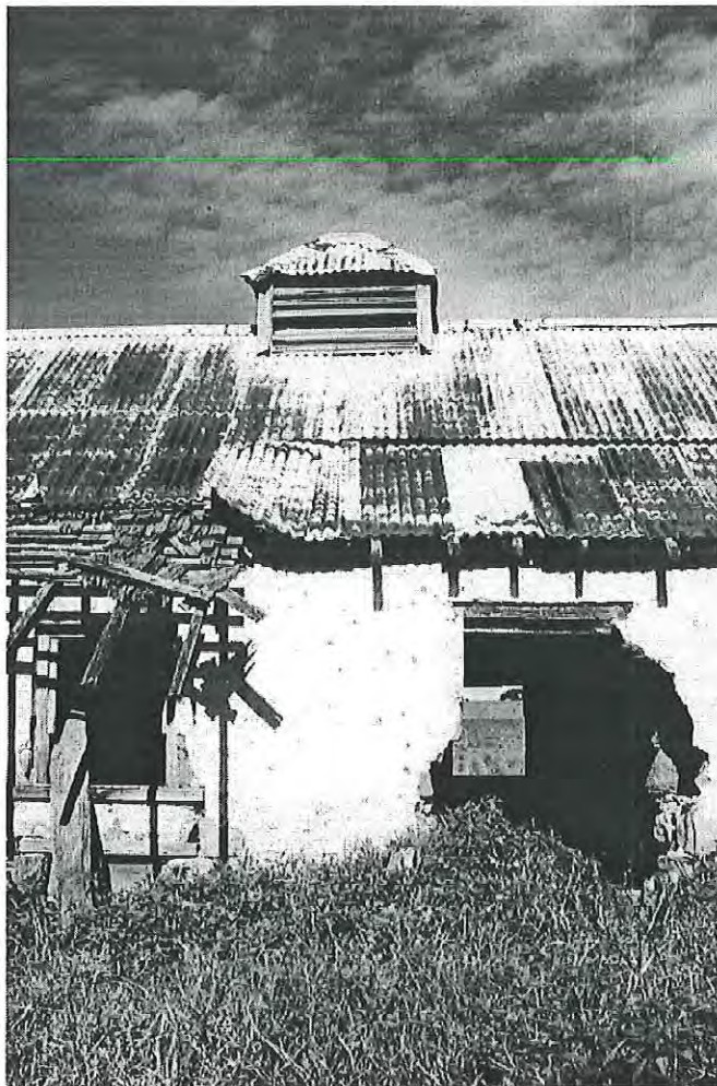
Below: Dairy interior, 70 cm thick walls rendered with mud mortar and whitewash; ventilation panels below windows, timber lintels; exposed timber lathes and underside of roof ventilation shaft as well as the vertical shaft of the collapsed eastern room ventilation shaft. Looking east MH 1997 photograph 10.16
