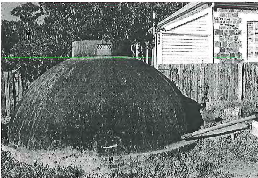
Dome top brick and render well similar to Mimosa Farm. MH 1997 photograph 12.9
