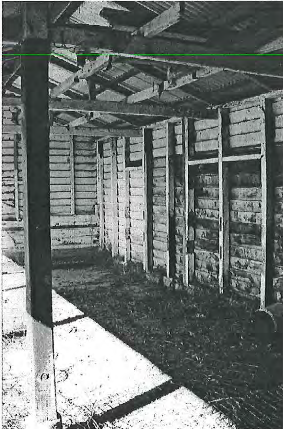
Above: Milking bails area, bails and milking machines removed and walk-through doors have been boarded up. Looking south-east. MH 1997 photograph 8.18
