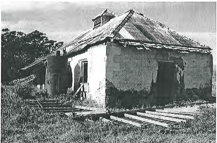
Dairy, rubble stone with roughly formed quoins, rough cast render with the quoins delineated in the render. Render washed away indication flood and rising damp levels. Collapsed verandah roof exposing shingles and shingle battens. Roof ventilation shaft, the eastern equivalent has collapsed. Riveted vertical boiler. Looking east MH 1997 photograph 10.14
