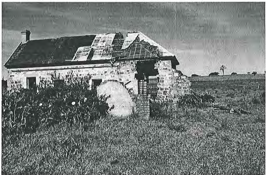
House - stone rubble roughly coursed, exposed shingles and remnant verandah fixture. Northern wing collapsed, ridge pole lying on ground RHS. Northern wing was keyed into a western hip extension of the original house. Looking south MH 1997 photograph 10.23
