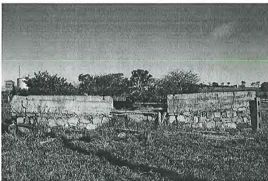
Sunny Vale. Feed stalls, stone rubble base, roughly coursed, concrete surface and formed walls lower section, 1918. Looking south MH 1997 photograph 11.11
