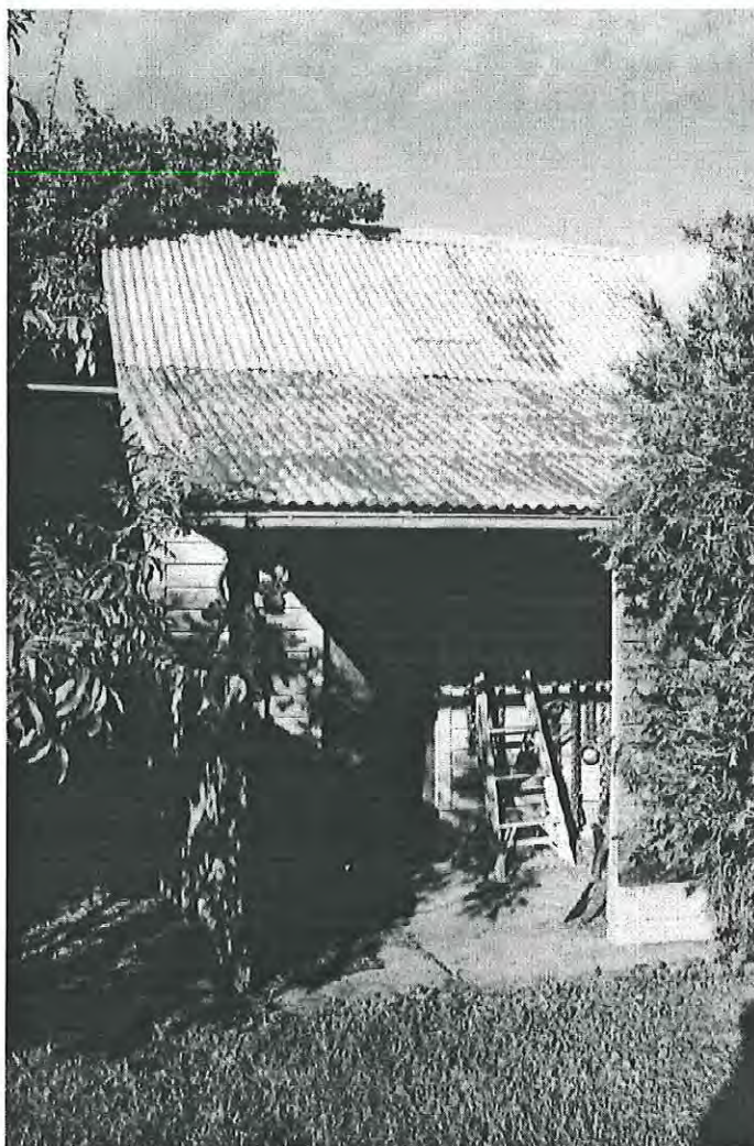
Right: Original dairy (creamery), hardwood weather board, early circular saw marks. Timber name plate above dairy door 'E (Elizabeth) Wood' - Registered Dairyman'. Looking south-east MH 1997 photograph 1.6
