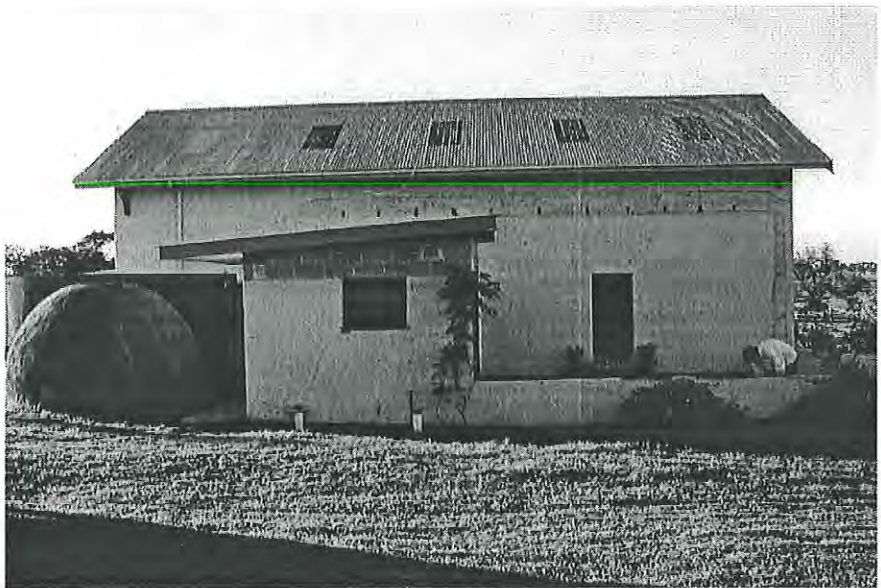
Southern elevation dome topped well, recent conversion of southern room to toilet block. Cool room walls reduced to dwarf wall height. MH 1997 photograph 13.16
