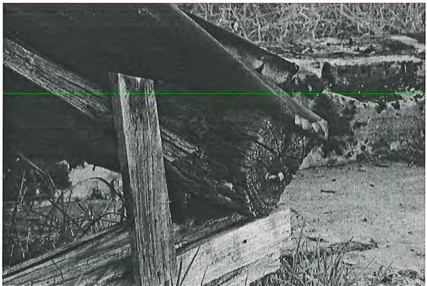
Detail of timber pegs used in construction of milking bails. MH 1997 photograph 14.7
