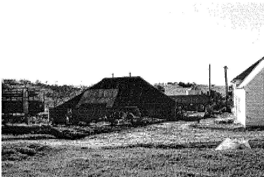
Dairy southern elevation showing alteration to roof to provide access to recent double garage doors. Looking north MH 1997 photograph 13.2
