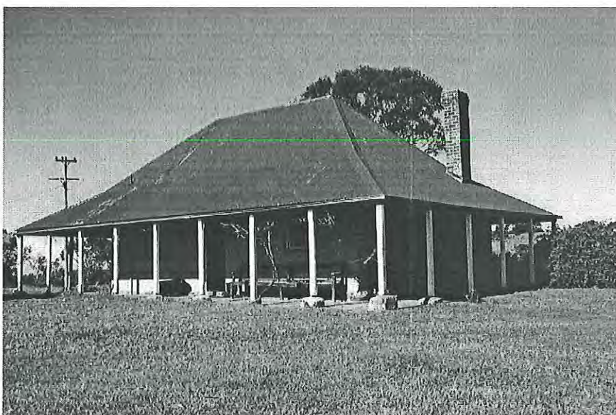
Narrawilly, early house, used as dairy (creamery); now accommodation. Painted brick with encircling verandah, enclosed at rear, stone floor, Looking south- west MH 1997 photograph 2.10
