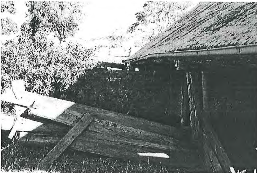
Eastern yards to pens, note drop log wall construction. Looking south MH 1997 photograph 12.14
