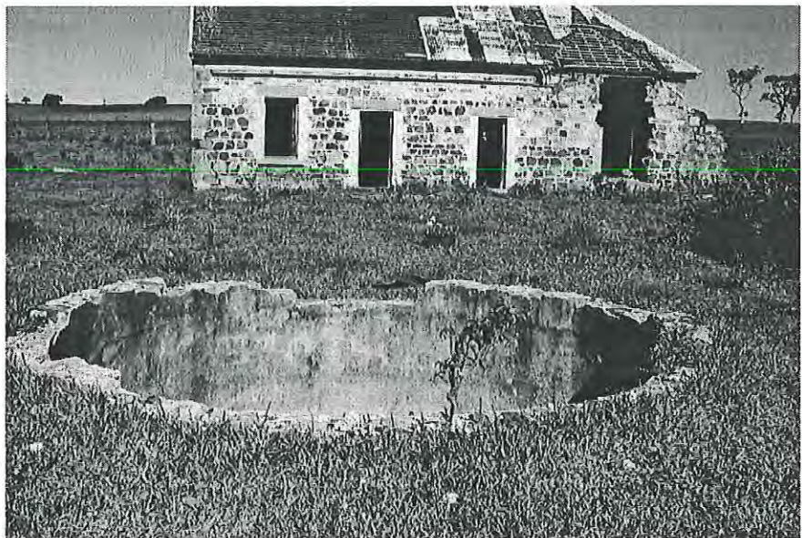
Brick and rendered well north of house. Looking south MH 1997 photograph 10.18
