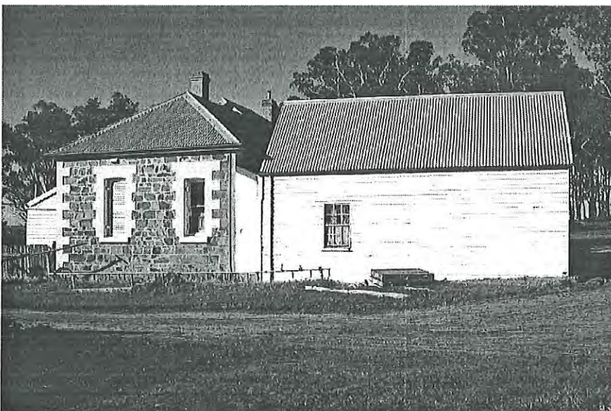
House western elevation, coursed random rubble with rendered quoins, shallow eaves, weatherboard pavilion extension with vertical board infill.. Looking east MH 1997 photograph 12.15
