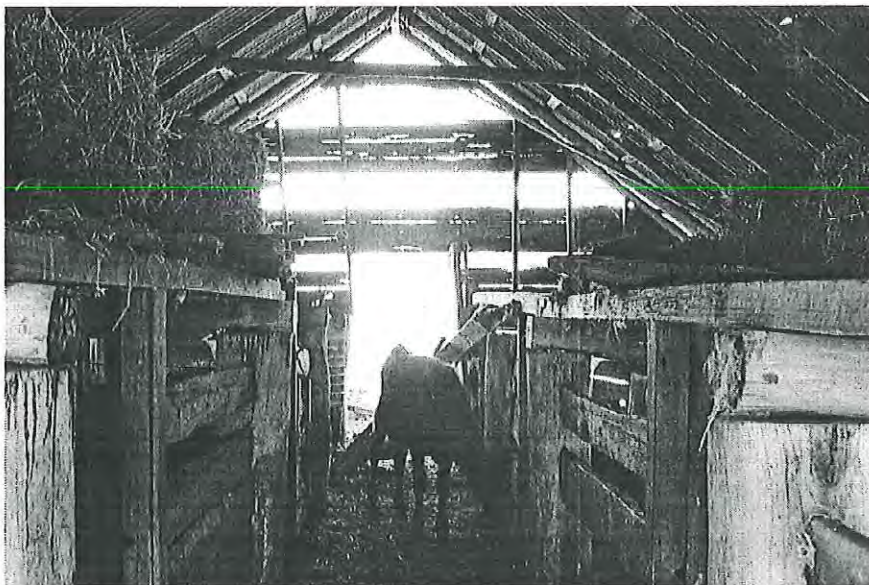
Pig sty interior central aisle, four stalls either side, over pen loft storage for fodder. Looking south MH 1997 photograph 12.12
