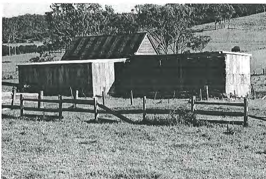
Large timber frame, corrugated iron hay and feed storage, post and triple rail timber fence. Looking south-west MH 1997 photograph 11.15
