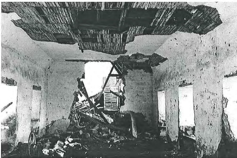
Below: Dairy interior, 70 cm thick walls rendered with mud mortar and whitewash; ventilation panels below windows, timber lintels; exposed timber lathes and underside of roof ventilation shaft as well as the vertical shaft of the collapsed eastern room ventilation shaft. Looking east MH 1997 photograph 10.16
