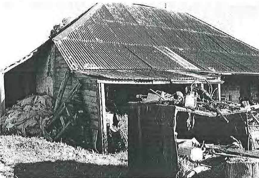
Northern Verandah extension to house engine to drive separator. Looking south-west MH 1997 photograph 12.3
