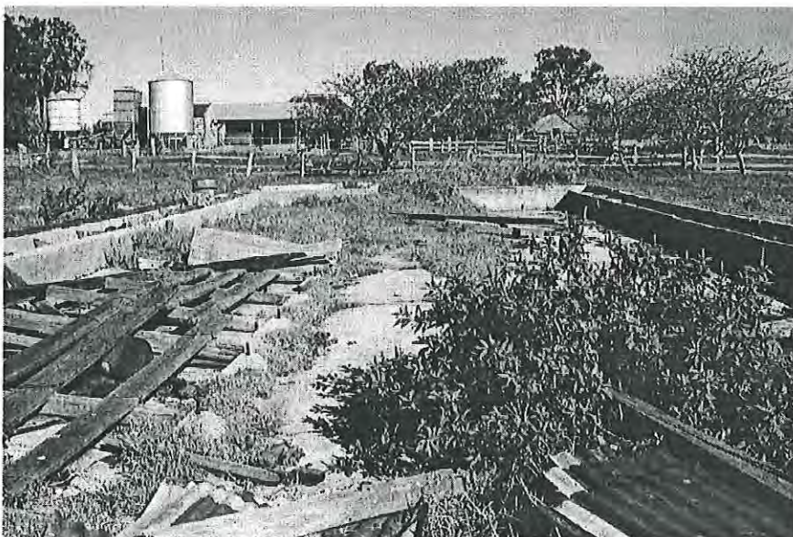
Feed stalls with formed concrete feed bins along outer walls, concrete plinths for timber posts as stall divisions, central aisle to feed storage areas at southern end. Looking south MH 1997 photograph 11.12
