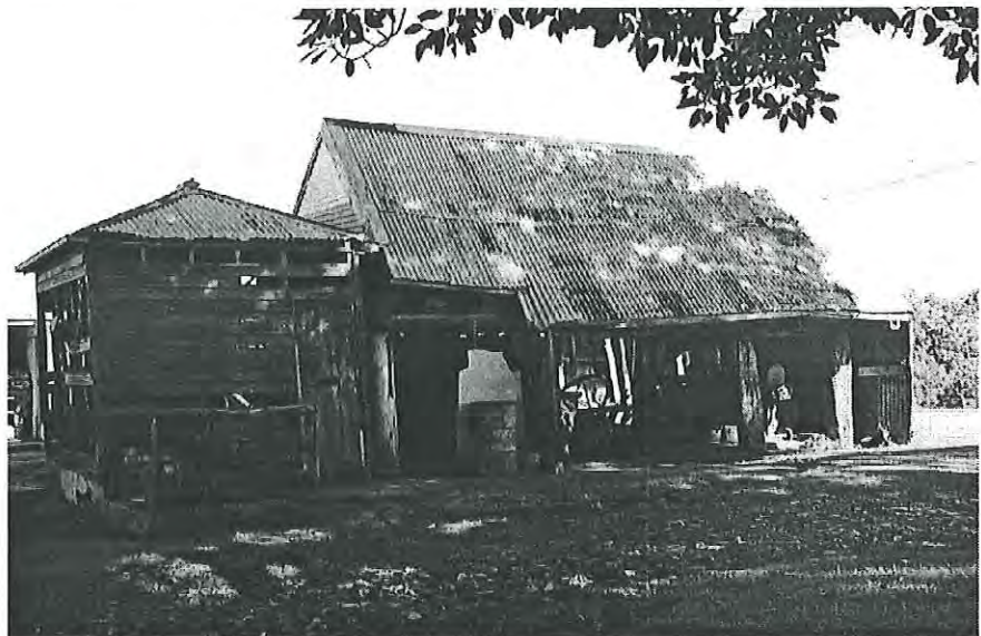
19th century bails. centre, engine room for milking machine, double up machine. Engine base extant. LHS, weather board milk can room with vertical board door. Looking south-west MH 1997 photograph 2 7
