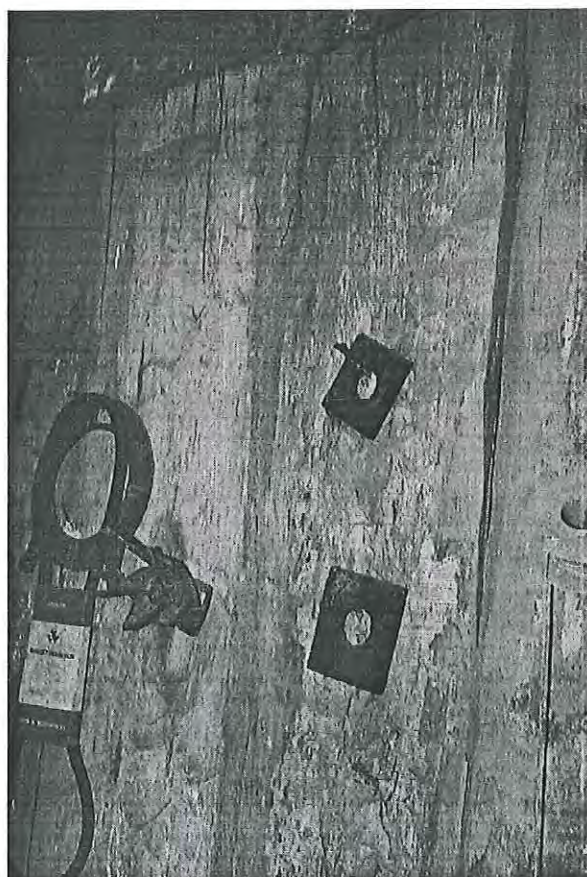
External slabs, residue newspaper. Looking south-east MH 1997 photograph 4.7
