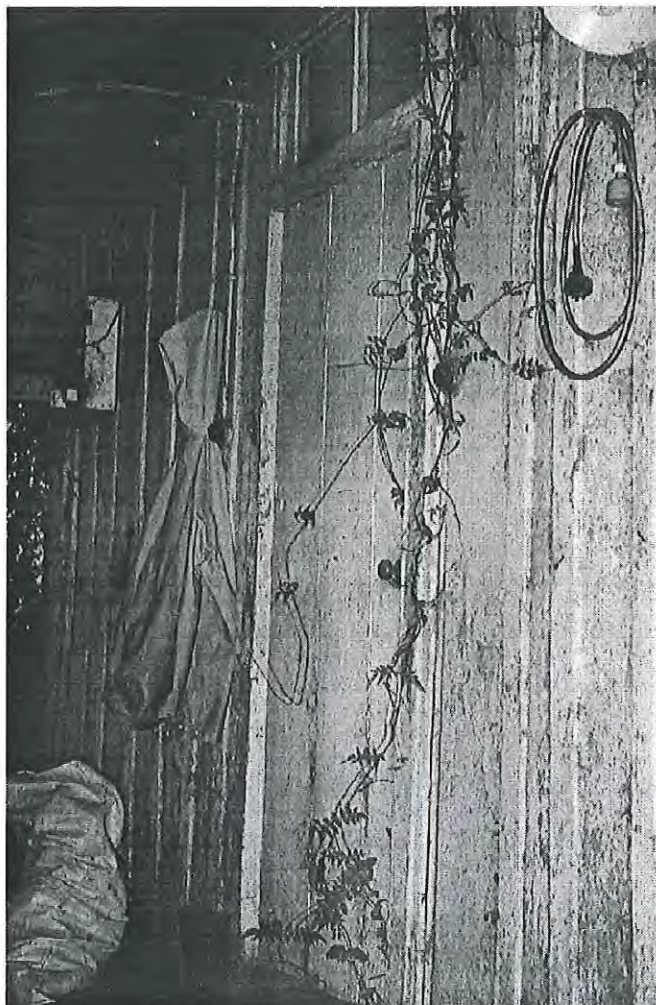
Right: Clinton Park. Mid 19th century slab and batten kitchen, chimney removed from eastern wall, skillion link to vertical sawn plank and batten house. Looking north-west MH 1997 photograph 7.3
