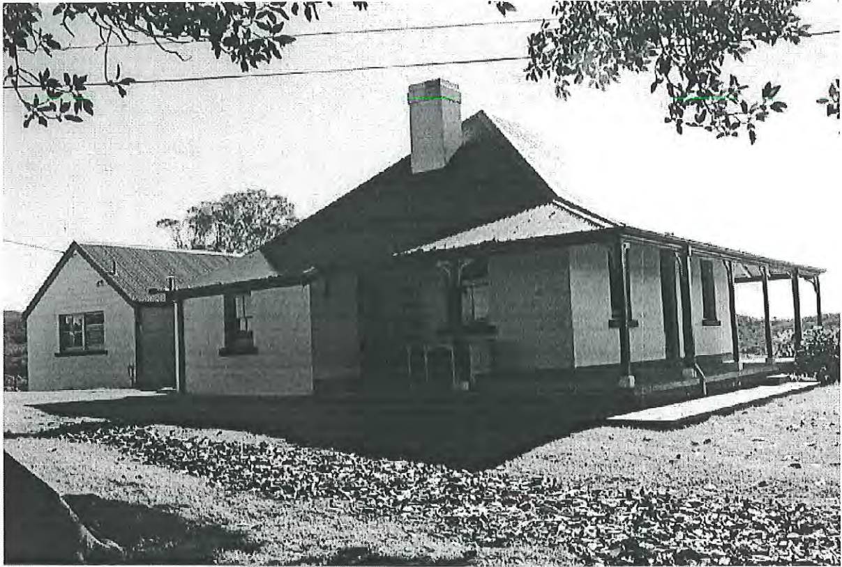
Woodlands house. Looking north-west. MH 1997 photograph 2 9
