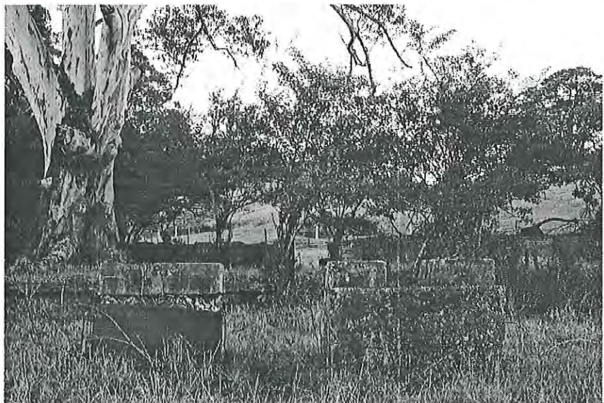
Concrete and aggregate plinths formed in ships water tank used to support shaft and flywheel between. Mounts have built in drainage funnel and drainage pipes for oil/water cooled bearings. Looking north MH 1997 photograph 7.22
