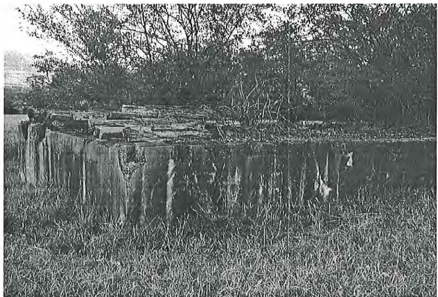
North eastern corner (refrigeration area, thick concrete base) showing recesses for joists extending north. Looking south MH 1997 photograph 7.25
