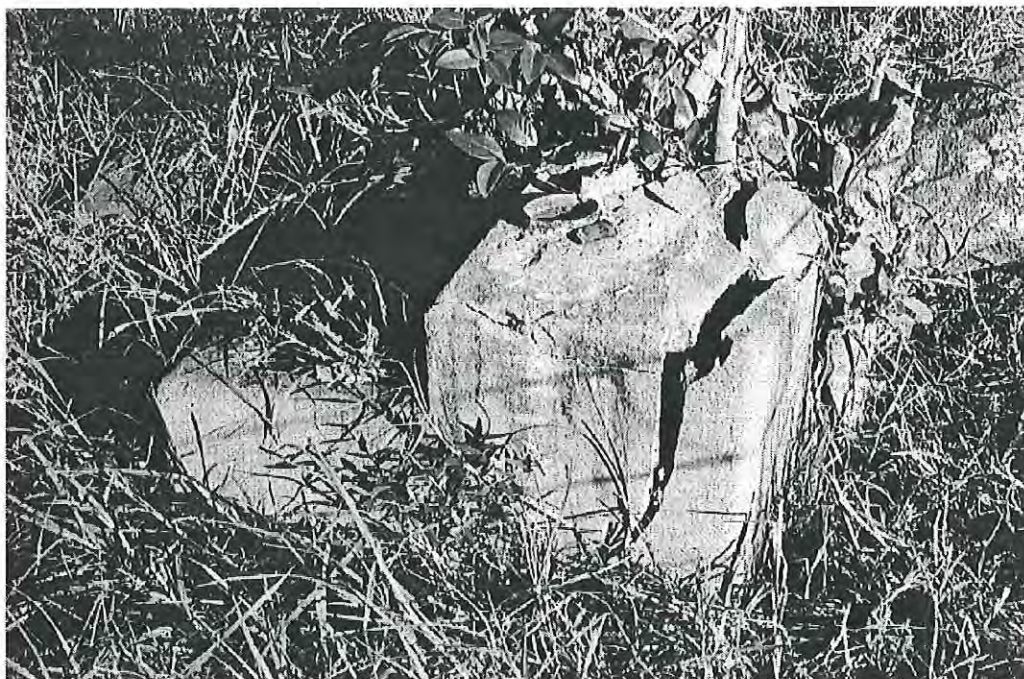
Below: Concrete plinth and pump mount and water trough adjacent to south of well, used for dairy purposes. MH 1997 photograph 9.12
