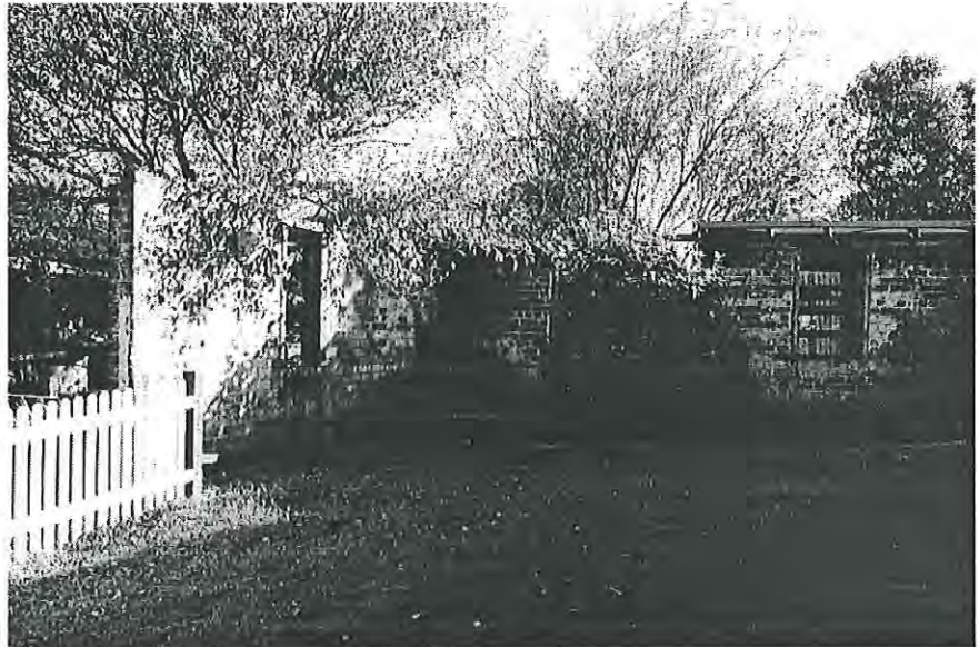
Remnant brick walls of earlier house/farm accommodation. Bricks similar to those made on site at Kendall Dale. Looking west. MH 1997 photograph 9.8
