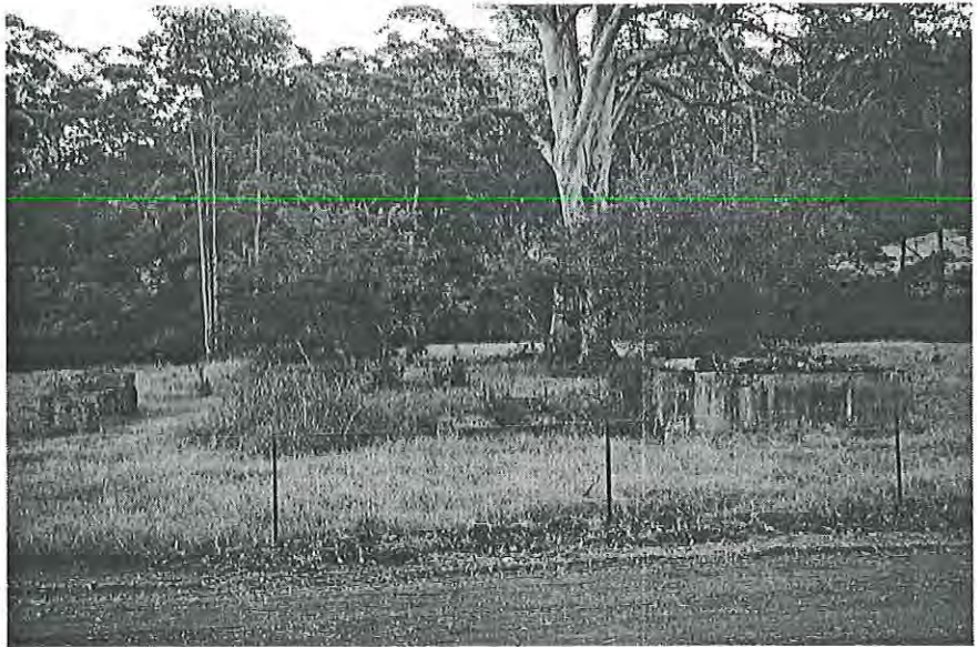
Barrengarry Butter Factory. Concrete foundations. Looking west MH 1997 photograph 7.20
