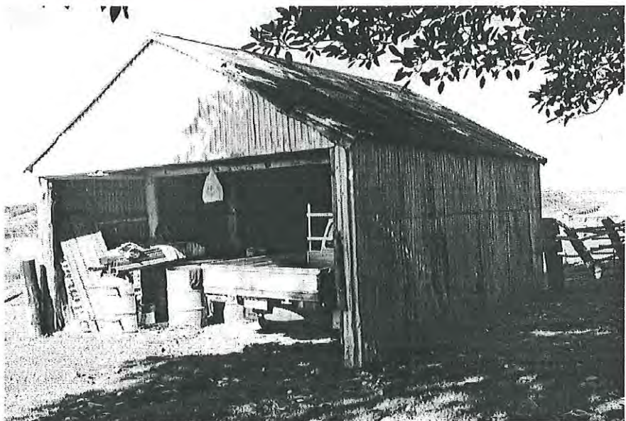
Garage, natural round posts, corrugated iron cladding, recent construction. Looking south-east MH 1997 photograph 2 8
