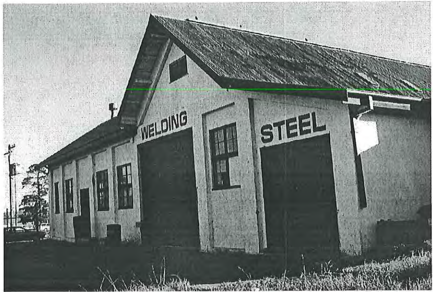
East elevation, wide eaves, louvre vent in gable, brick with cement render, pilaster architectural detail, 4x2 pane timber windows, surrounded by dish drain. Looking south- west MH 1997 photograph 3.9
