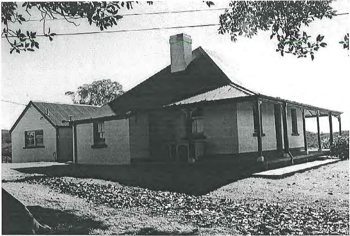
Woodlands house. Looking north-west. MH 1997 photograph 2 9
