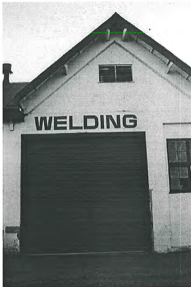
Right: East elevation, delivery receiving dock for milk to be processed. Dock has been cut to form doorway, later use of sit, ice works, fish processing, produce packaging. Looking west MH 1997 photograph 3.8
