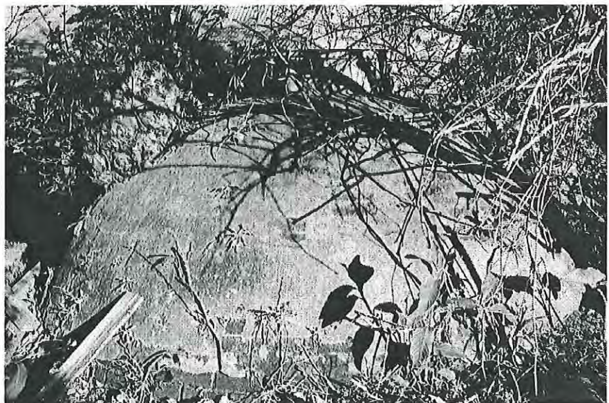
Cement rendered brick dome topped tank c.1880. Looking west MH 1997 photograph 9.11
