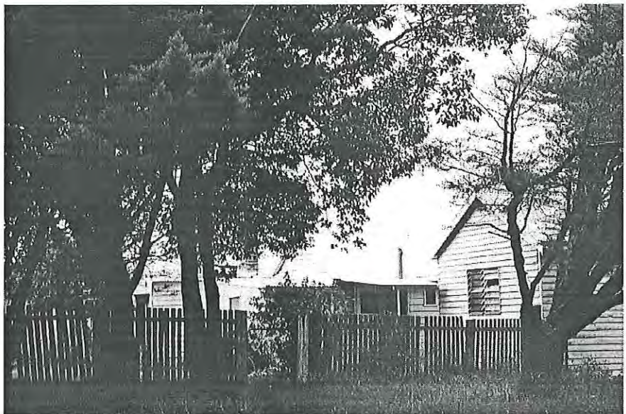
Timber picket fence & windbreak for back garden. Looking south-east MH 1997 photograph 3.20
