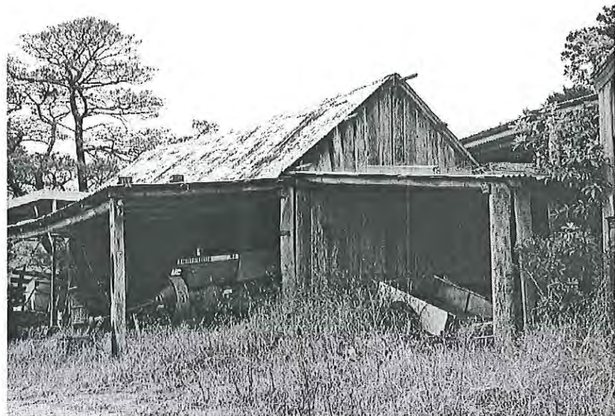
Corn shed and workshop. Looking south-west MH 1997 photograph 4.8
