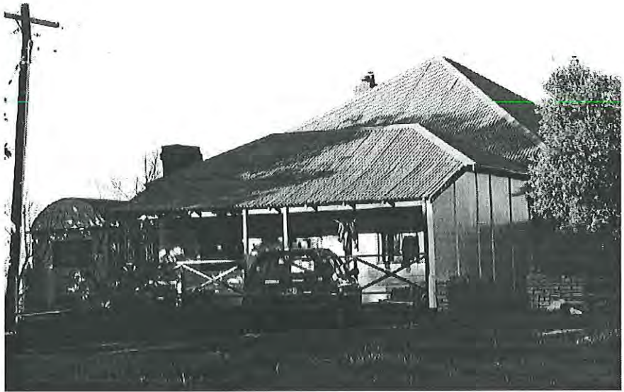
Western elevation of detached kitchen, early 19th century weatherboard construction, set off centre to central hallway in house, now connected to house through skillion. (Possibly relocated from elsewhere.) Looking north-east. MH 1997 photograph 9.20
