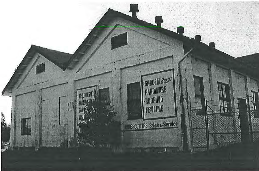
Above: Milton Butter Factory, Looking north-west MH 1997 photograph 3.4
