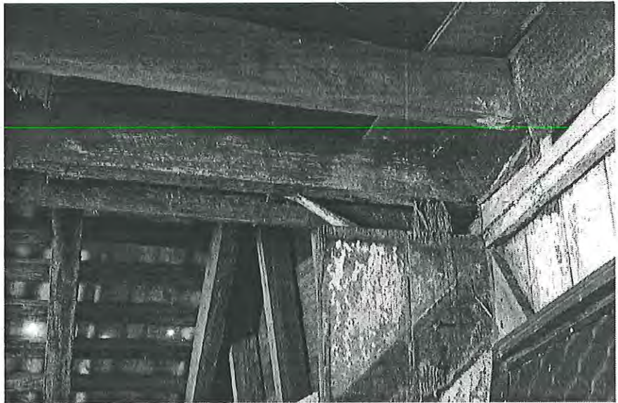
Detail of wall and roof construction, shingle battens in situ. MH 1997 photograph 9.16
