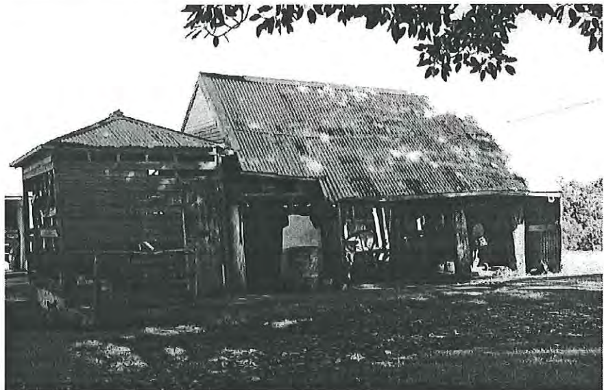
19th century bails. centre, engine room for milking machine, double up machine. Engine base extant. LHS, weather board milk can room with vertical board door. Looking south-west. MH 1997 photograph 2 7
