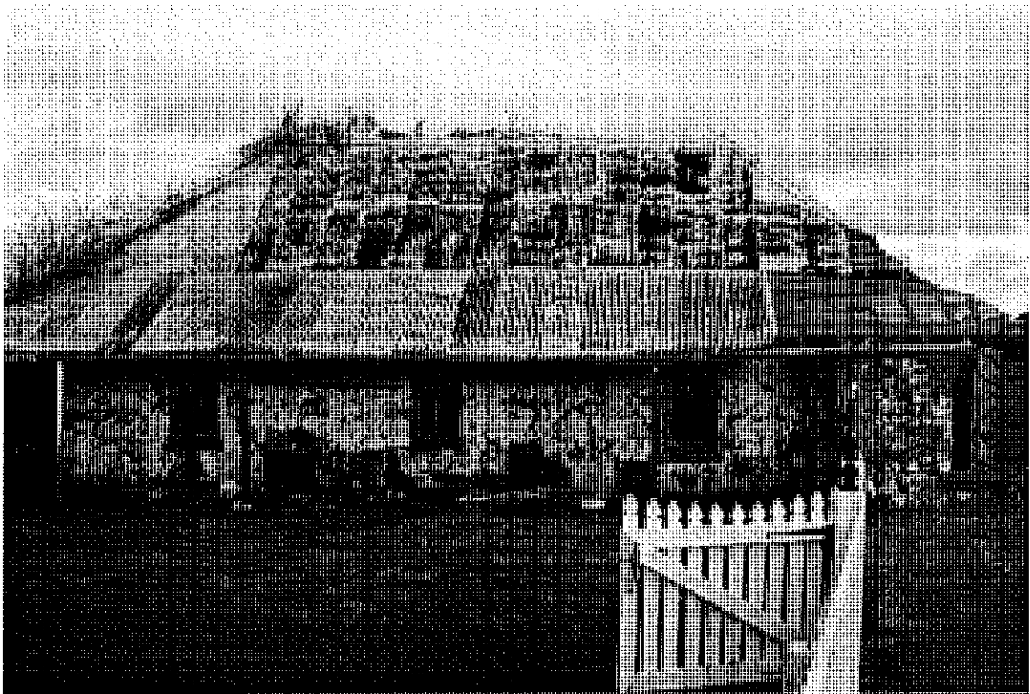
Above: 'Avenal', early kitchen, random local stone and mud mortar, scullery addition to. Kitchen and Maids room. Scullery chimney in brick, kitchen chimney in stone. Looking east. MH 1997 photograph 1.9
