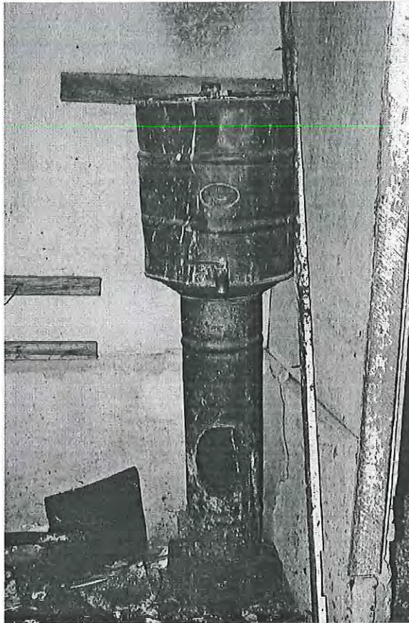
Moorehouse the Machinery Man, Nowra, hot water heater, typical of south coast dairies. MH 1997 photograph 4.16
