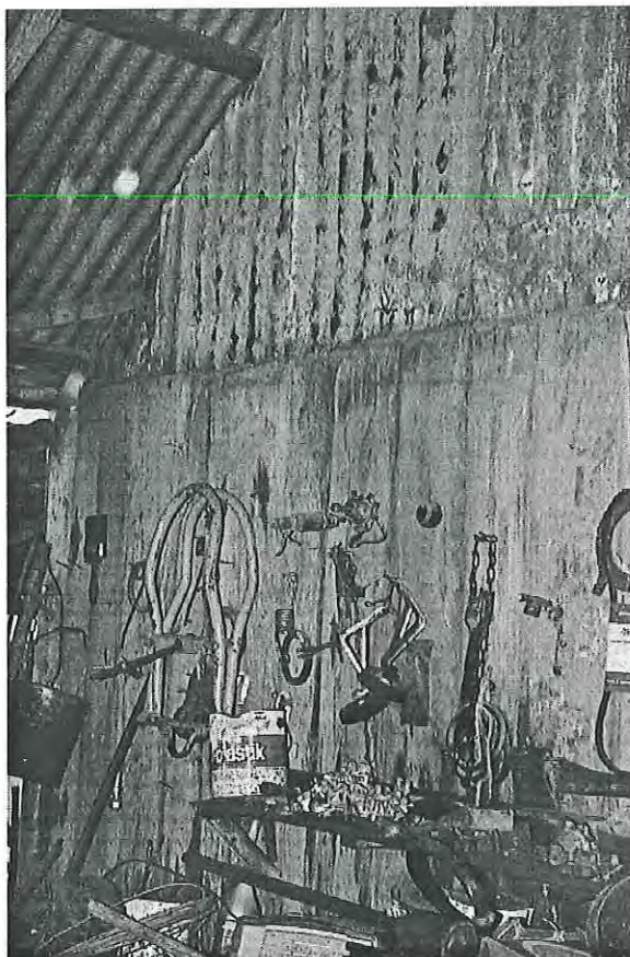
Detail of timber construction, corn store, external north, slabs nailed onto round timber frame. wall now covered workshop. Looking south-east MH 1997 photograph 4.6
