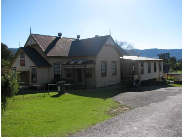
Community Hall with parking area in foreground
