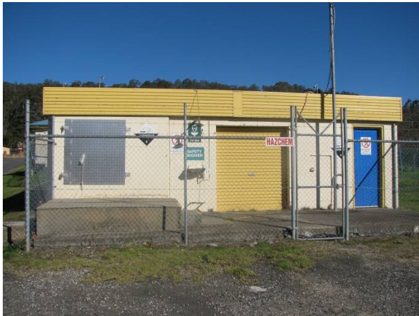
Machinery and chemical storage building
