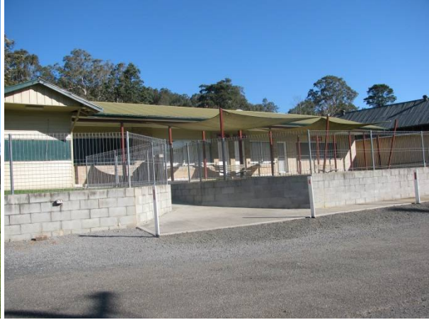
Building with access ramp and retaining walls adjoining access road
