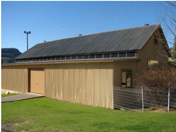
Agricultural Pavillion – Viewed from Community Hall side
