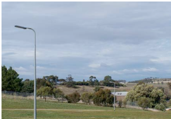
T5 luminaire after installation
