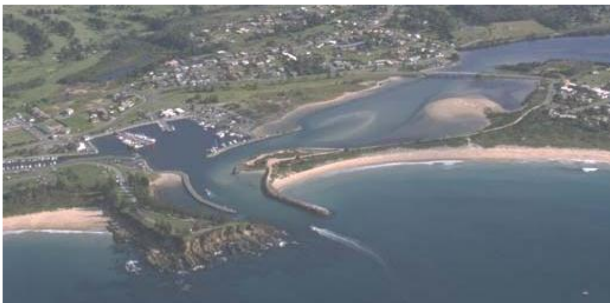
Example of breakwaters at Bermagui showing general scale of works
