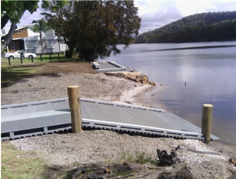
Photo 4 Milham Street Foreshore Rehabilitation
