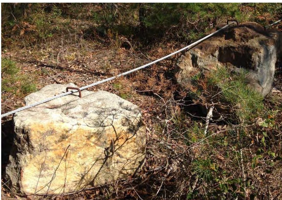
Plate 3 - A rock and cable fence, typically used where bedrock hinders installation of posts
