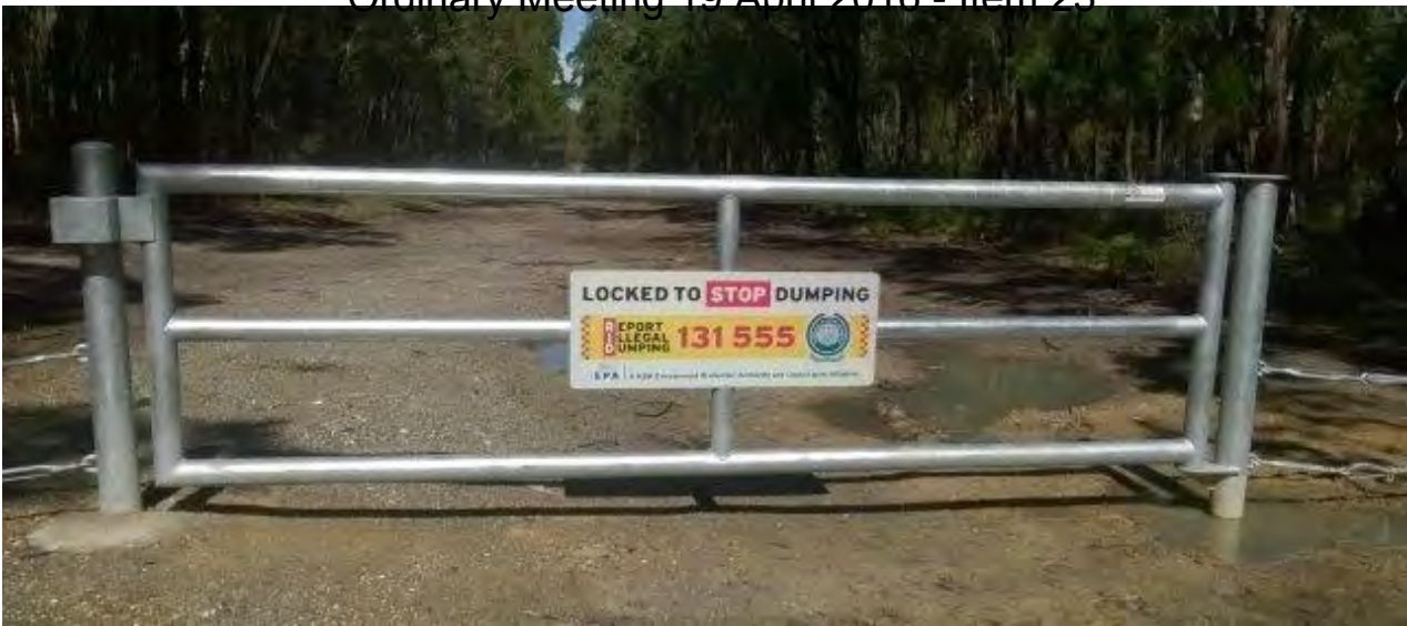
Plate 1 – Photograph of a gate installed along Forest Rd. This is the style of gate proposed at both ends of Birriga Ave and the southern end of Wanawong Bld.
