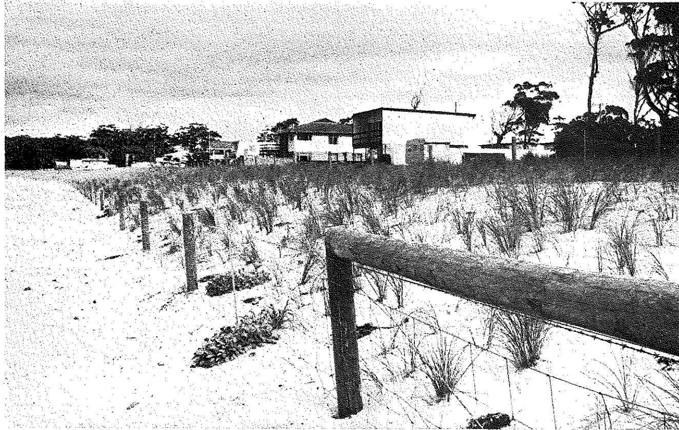
Figure 7—Southern end of restoration works, six months after implementation of the scheme.
