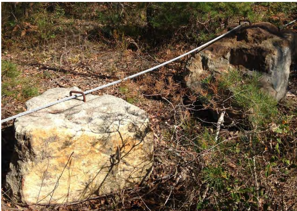
Plate 3 - A rock and cable fence, typically used where bedrock hinders installation of posts
