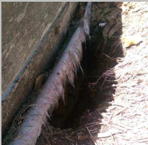
Photo 32 Erosion behind retaining wall
