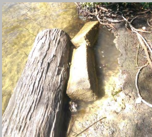
Photo 29 Displacement of Protection
