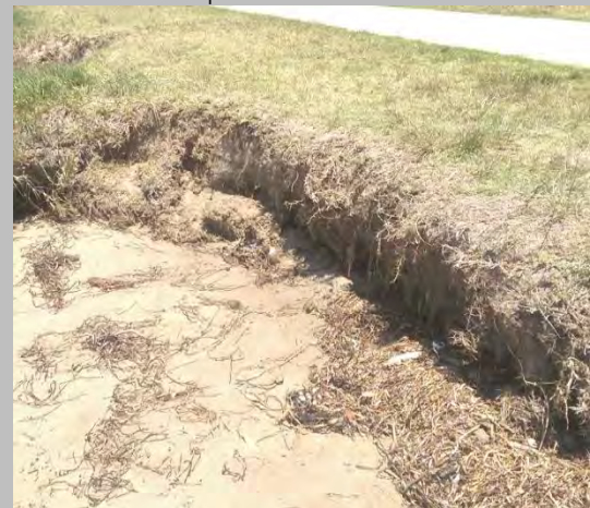
Photo 12 Exposed bank erosion
