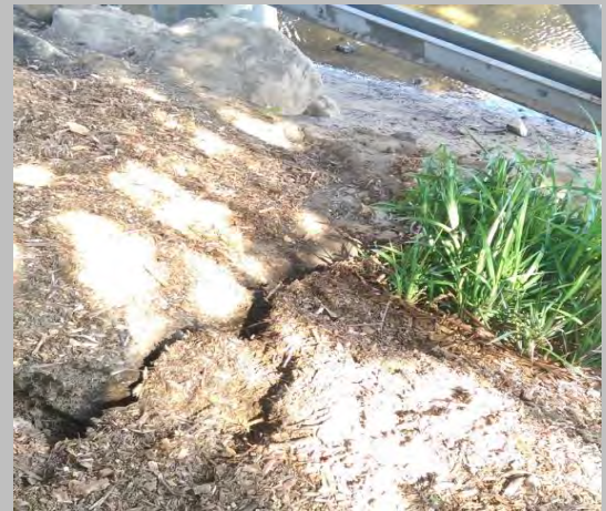
Photo 4 Erosion behind revetment
