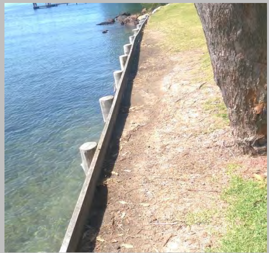
Photo 33 Timber Retaining Wall
