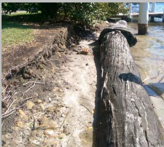
Photo 28 Displacement of Protection
