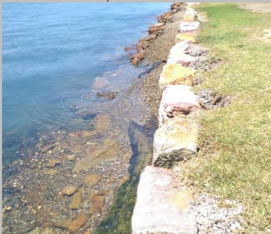
Photo 11 Toe protection failure
