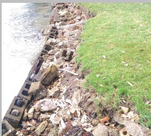
Photo 39 Erosion behind protection
