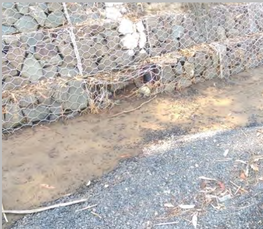
Photo 3 Damaged Gabion Mattress
