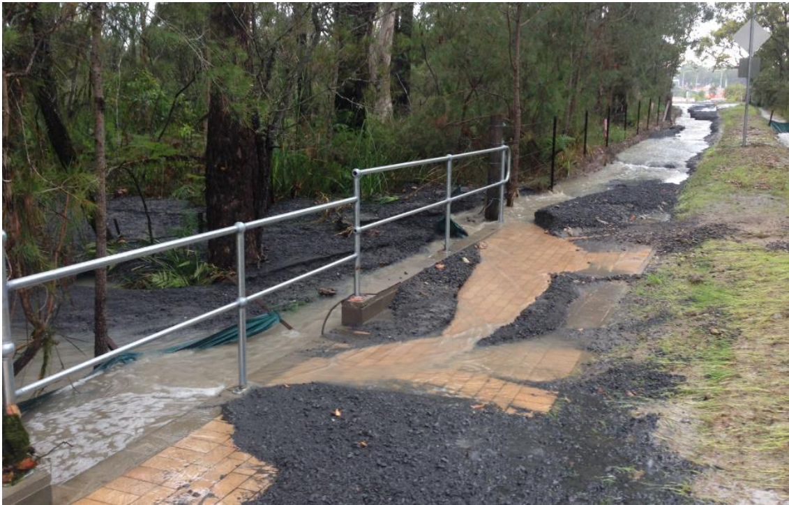
Figure 2 – Paved Area (With gravel deposition shown on the pathway and in the adjoining natural area.)
