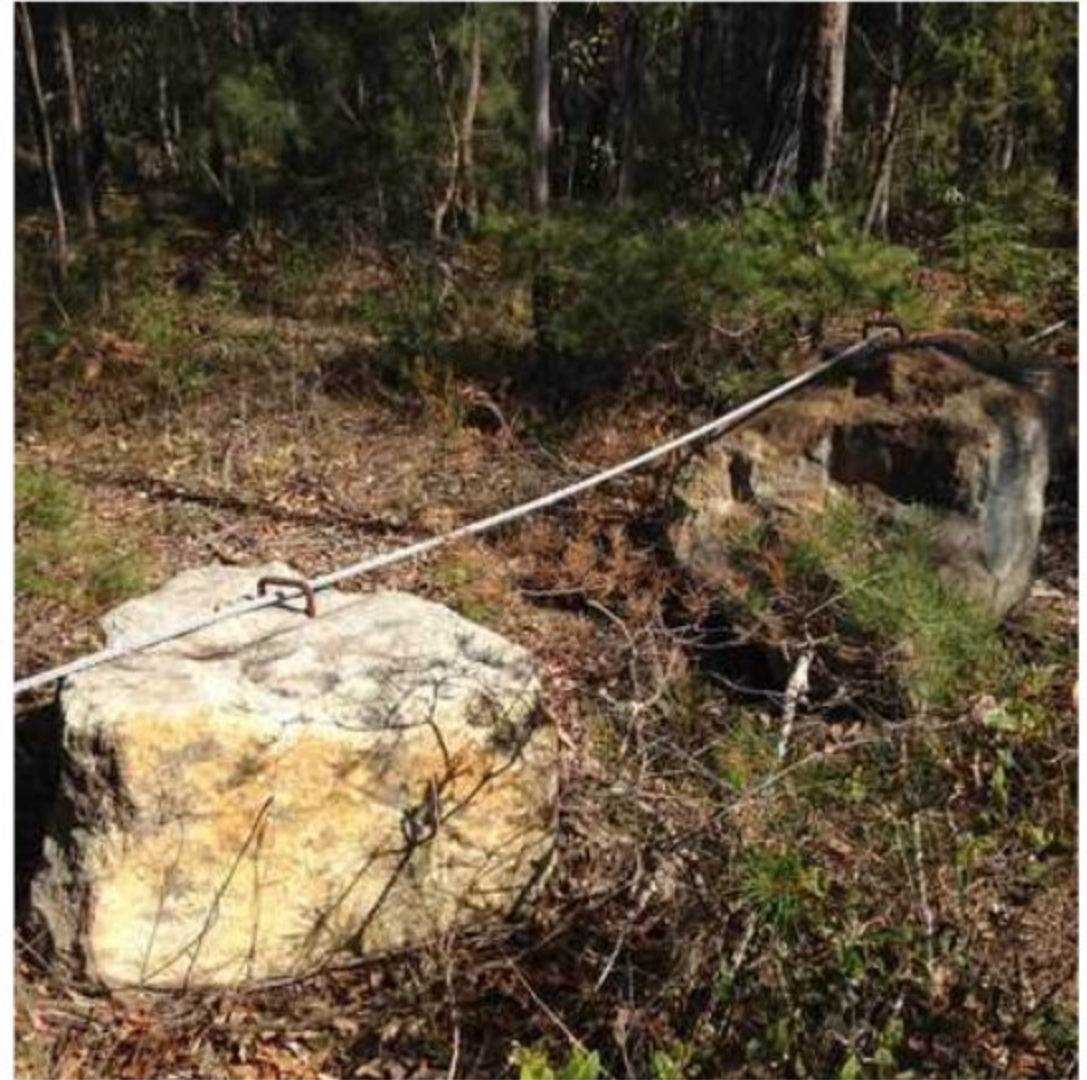
Example of Cable & Rock Fencing
