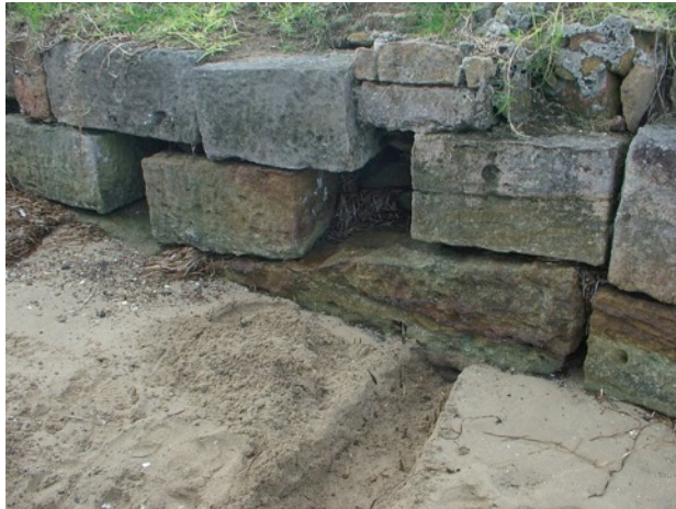
Figure 3.12: View of Wall 1 in July 2006 with concrete rubble repairs in the top right corner of shot, looking north (Source: Cosmos Archaeology).
