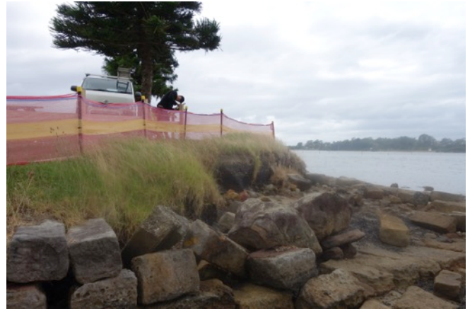
Figure 3.8: Wall 1, in foreground, in December 2015 looking north. Shows little or no movement of the dislodged blocks since 2006. Also the grassed bank in the foreground seems to have encroached on the blocks of Wall 1 while the same bank in the background seems to have receded slightly. (Source: Cosmos Archaeology)
