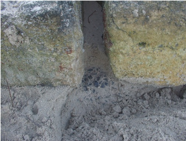
Figure 3.22: Wall 3 in July 2006. Sandstone blocks sitting on lower course of concrete with bluestone aggregate. (Source: Cosmos Archaeology)
