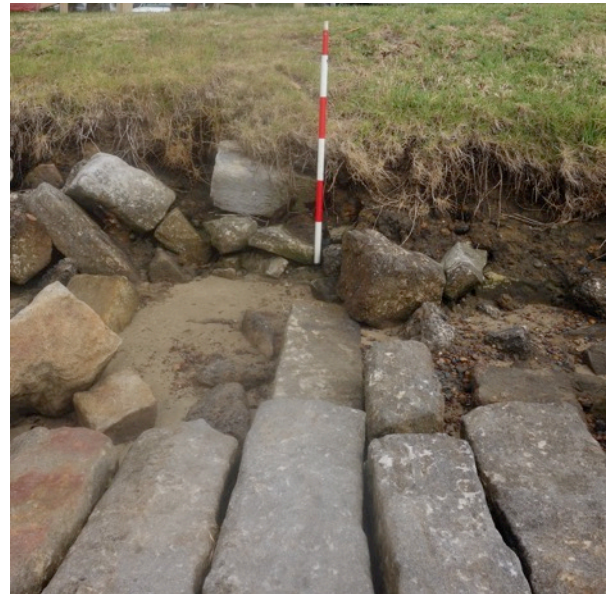
Figure 3.21: Wall 3 in December 2015, looking west. Note the reduction of sand levels between the wall and the grassed bank – ca. 0.25 to 0.40 m. The bank itself has slightly eroded –perhaps by 0.25 m. Scale in 200 mm increments. (Source: Cosmos Archaeology)
