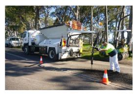
Heavy patching does require more resources and planning than a pothole repair. So, the pothole repair many be implemented initially to manage the hazard, while the heavy patch can be designed and programmed.
