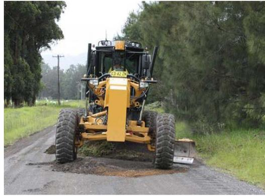
**Termeil - Old Princes Highway - Works involve a low cost seal, consisting of a pavement over lay and bitumen seal. Works will be undertaken between the existing seal and #295. The works have commenced and are scheduled to be completed by 21 July.**
