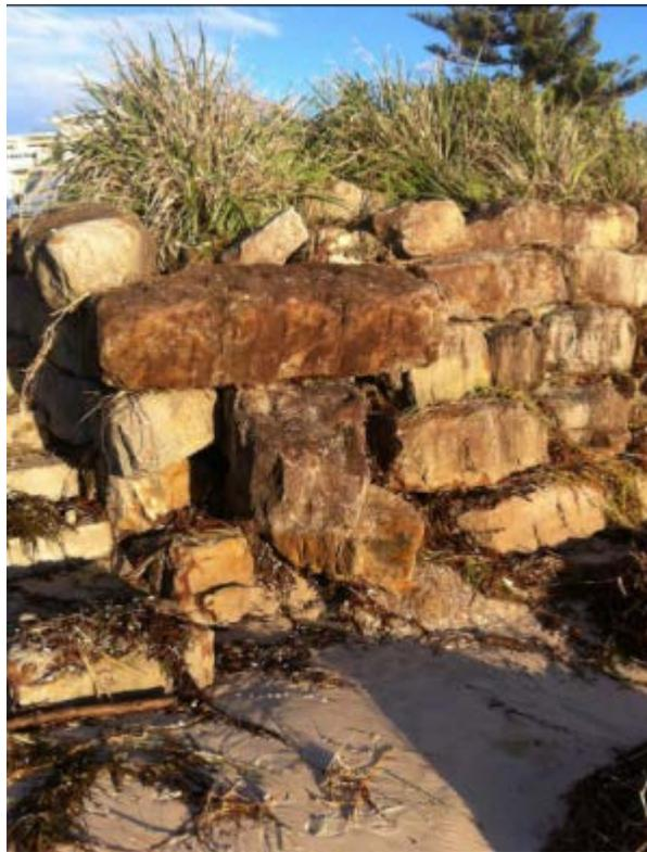
The sandstone block wall partially collapsed as a result of the June 2016 east coast low storm.
