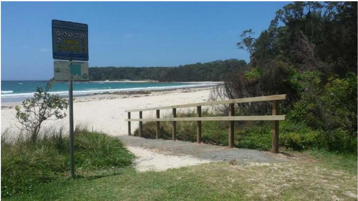
Washerwomans Beach Bendalong - the ramp and handrail replaced a step off an erosion scarp onto the sand.
