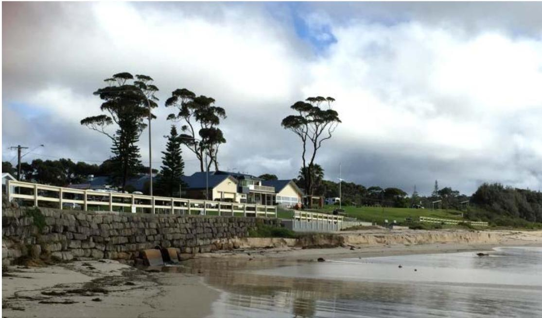
The 1974 storm also destroyed part of the road at the corner of Golf Avenue and Ocean Street, just behind the sandstone block wall (shown above). It was soon after this that the sandstone wall was constructed. The wall was 'not designed to resist major storm wave attack and.....the size of the rock is inadequate.' Public Works Department 1987.
