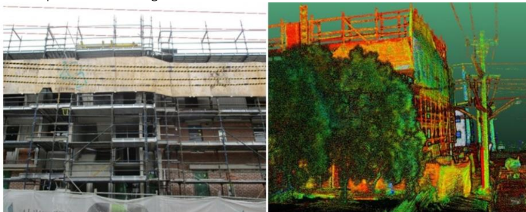
Image 1 (left): Construction site where work was being done – noting red lines indicate where the power lines were located. Image 2: (right) Lidar scan image, showing construction site and power lines where work was being done.
