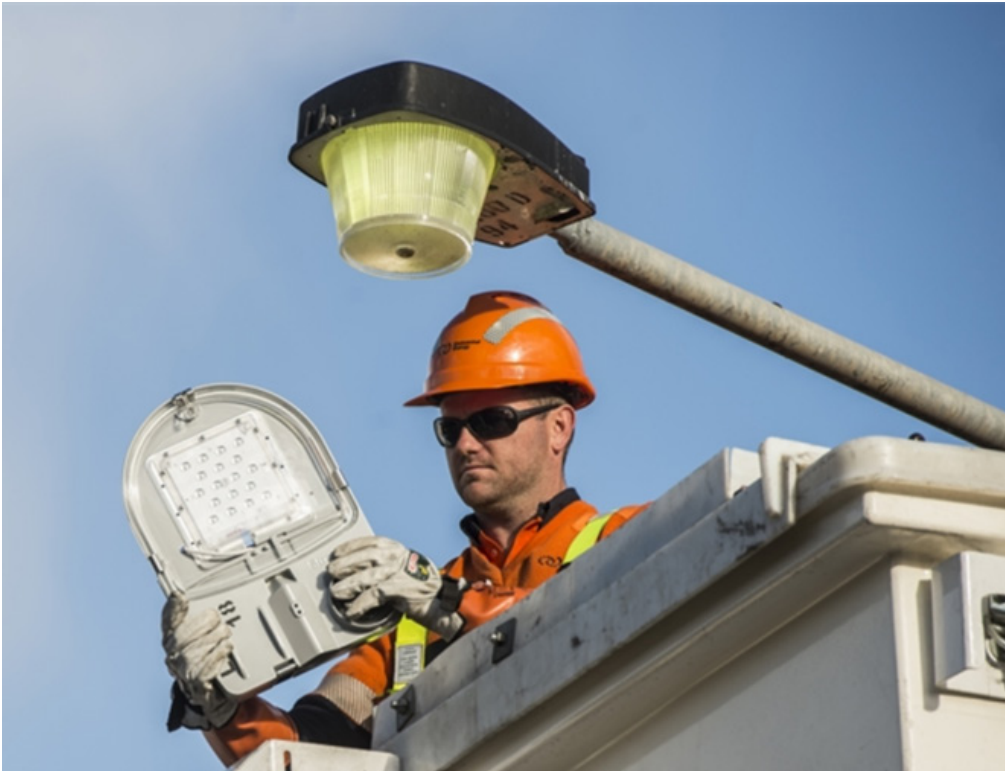
Supply of retail electricity for Council's large sites and street lighting
