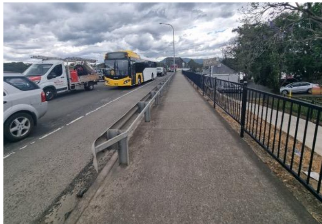
Figure 39: Narrow footway at Nowra Bridge alongside a heavy traffic creating a noisy environment (Source: CrossleyTP, 2022)
