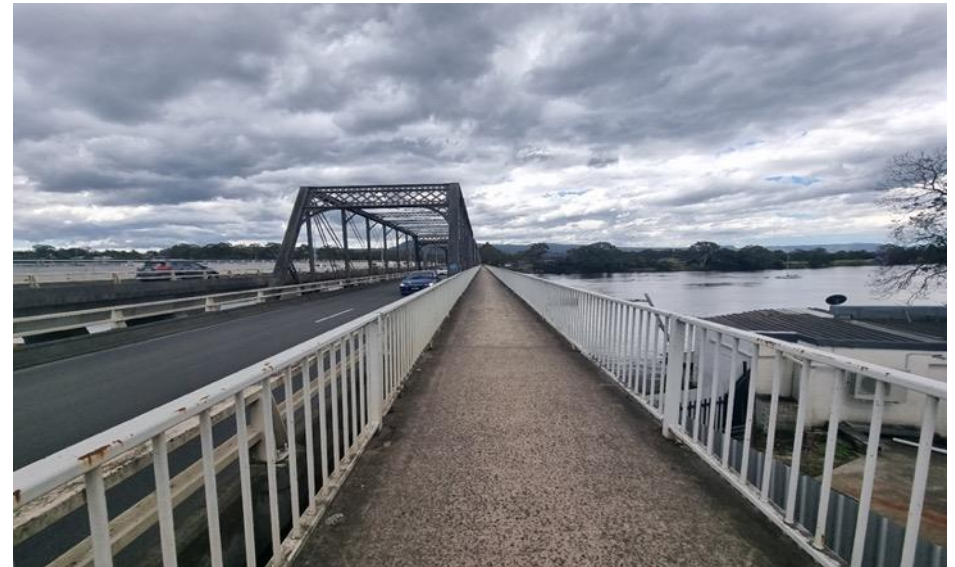
Figure 2: Shared User Path on the Nowra Bridge (Source: CrossleyTP, 2023)
