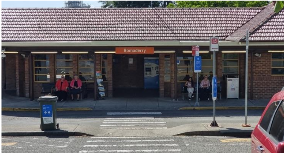
Figure 11: Bomaderry Station (Source: CrossleyTP, 2023)
