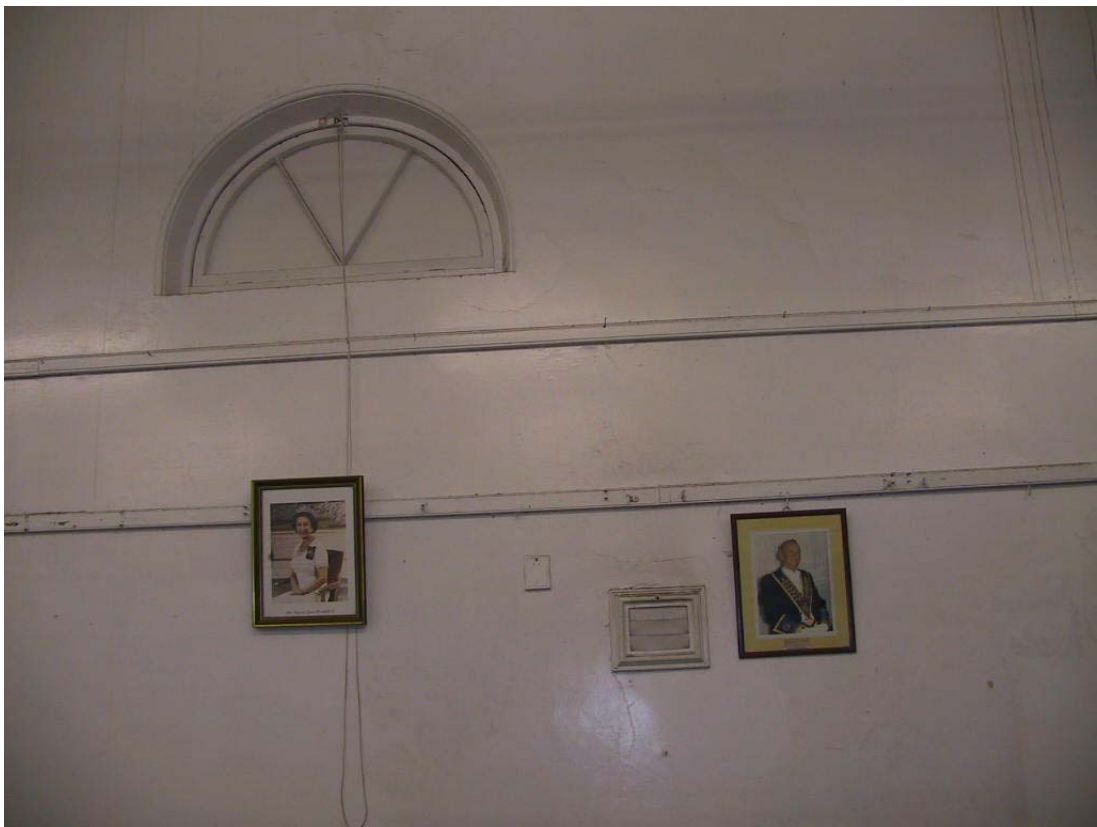
Figure No.33 & 34: Examples of typical semi circular windows and picture rails located in the Lodge room
