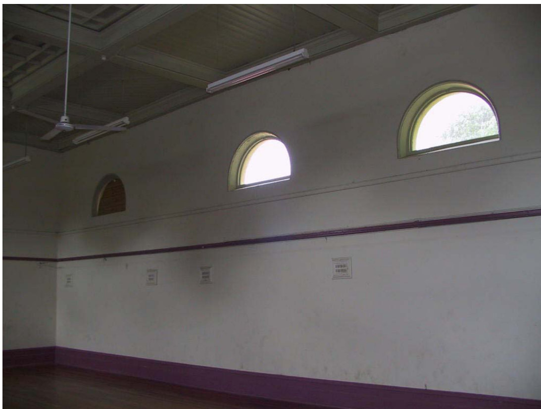
Figure No.42: The Supper room looking towards the east.
