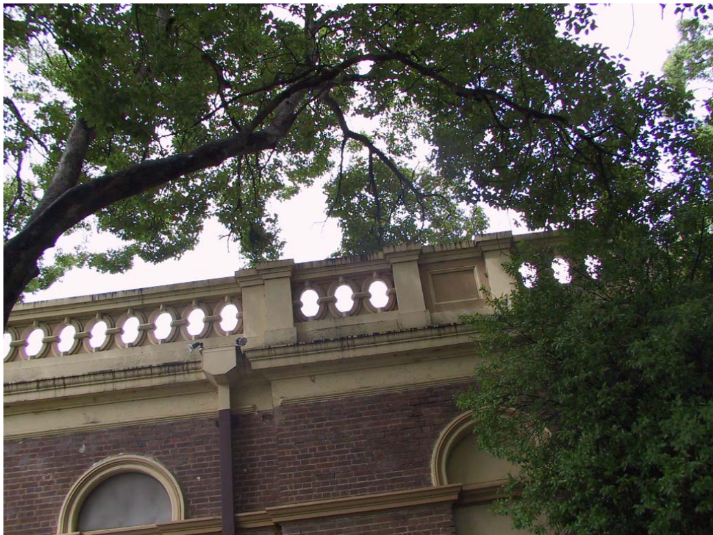
Figure No.19 & 20: The subject building showing the parapet
