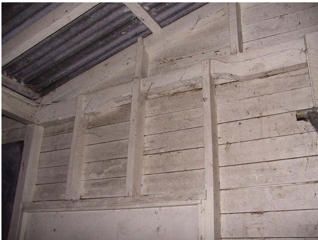
Figure No.48: The servery area of the rear addition.
