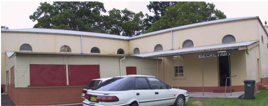
Figure No.10: Rear elevation of subject building
