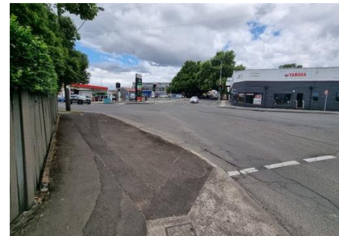
Figure 38: Uneven pedestrian surface along Bridge road (Source: CrossleyTP, 2022)
