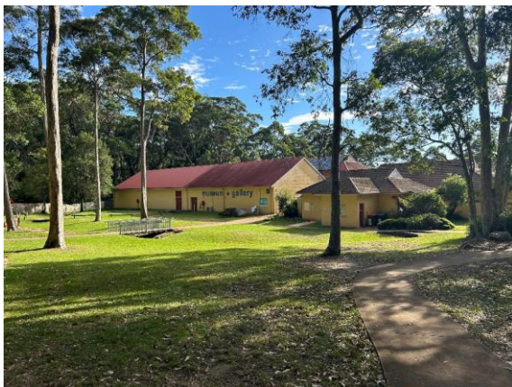
View looking north-east across drainage swale towards main entry to museum building
