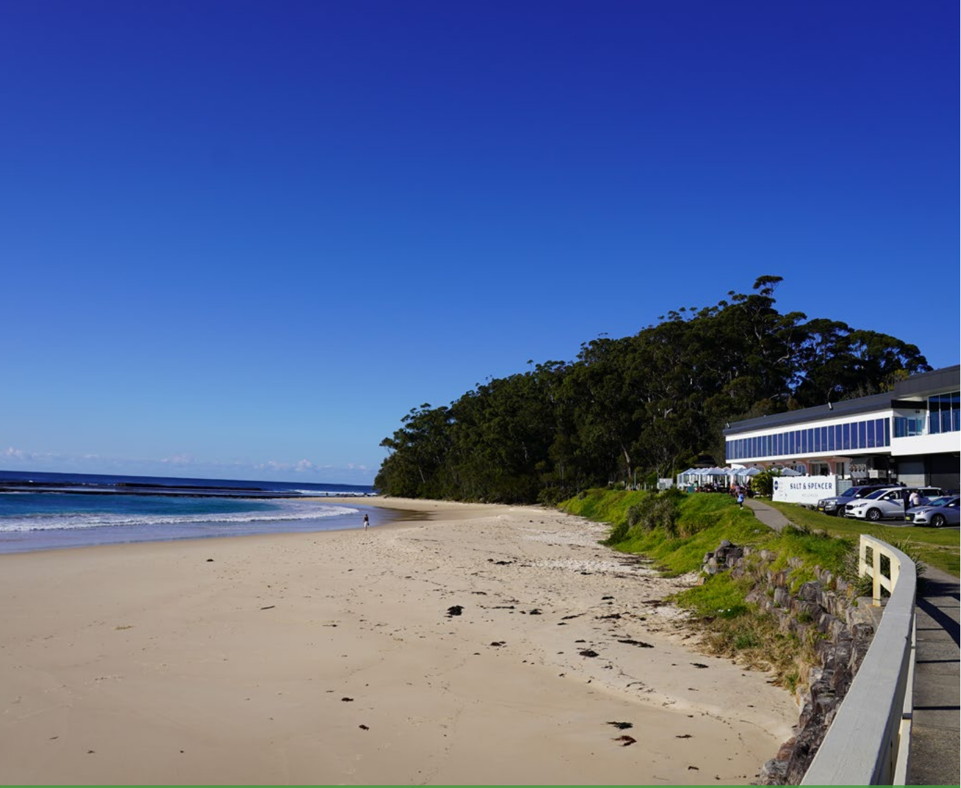
South Mollmook Coastal Protection works
