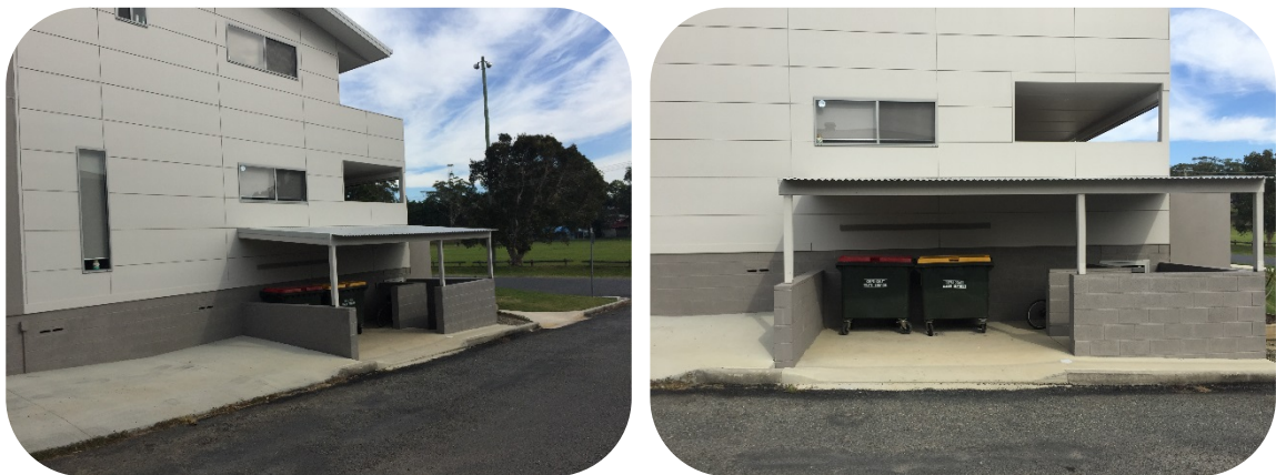
Figure 3.4 - Example of poor quality design of bin storage space added to outside of building with high street exposure, poor accessibility for residents and lack of adequate cleaning space.
