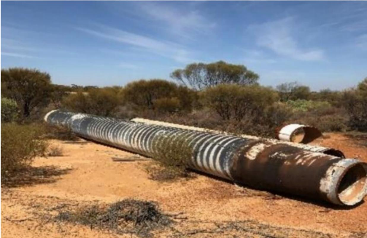
*Figure 22 - Weathered asbestos coal tar coated pipe at Boondi Pump Station. Note the spiral wrap and the remnant whitewash, especially on the underside of the pipe.*
