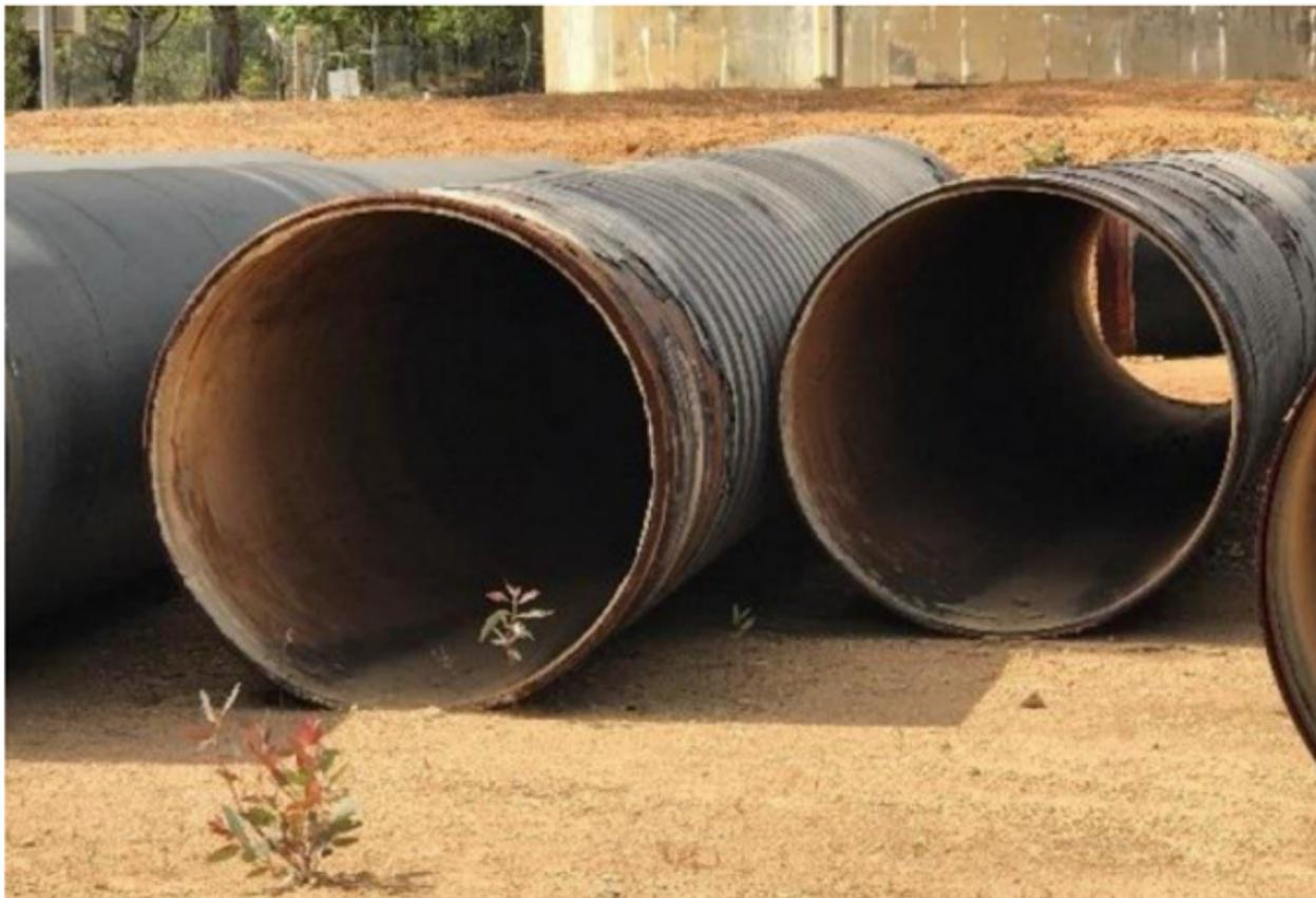
*Figure 28 - Weathered asbestos coal tar coated pipe at Fleay Road, Harvey. Note the spiral wrap, remnant whitewash and coating colour weathered to light grey.*
