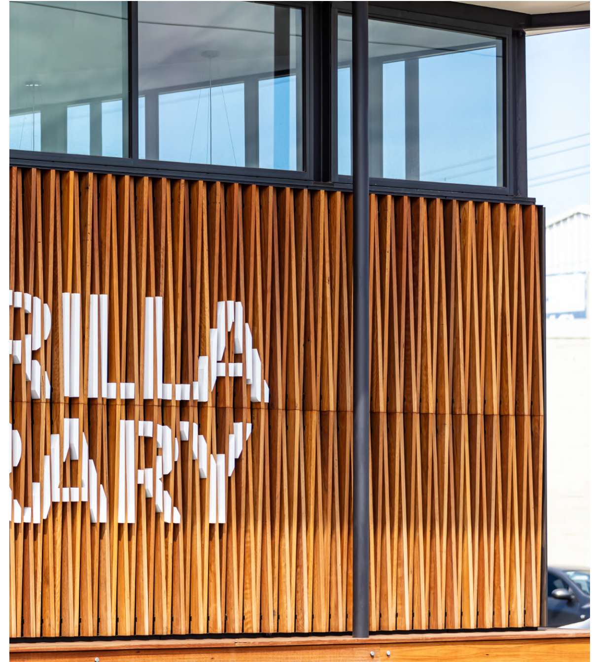
Detail photograph of timber batten facade at Warilla Library
