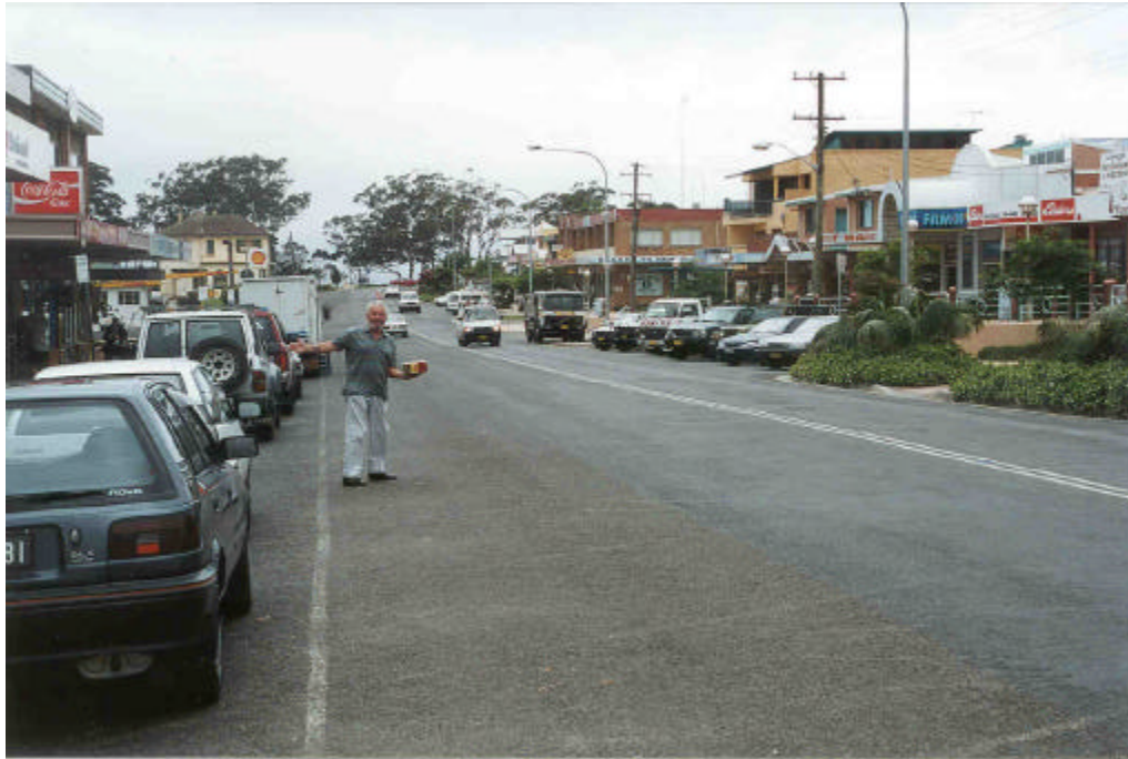
■ Photograph 15 – One-sided Kerb Build-out, Owen Street, Huskisson
